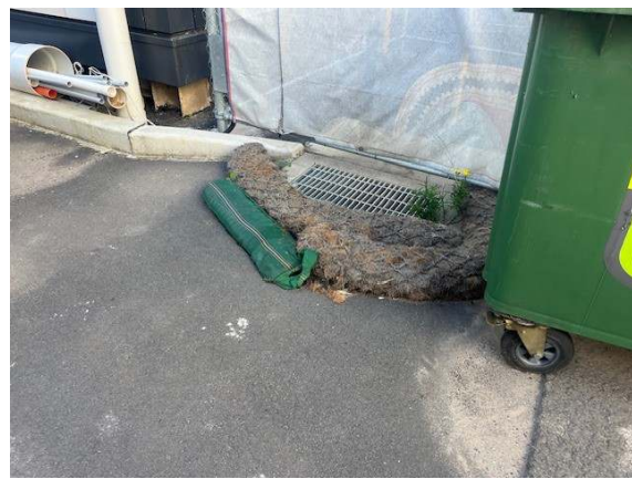
Photo 7: Controls in place around stormwater grates in the site compound.
