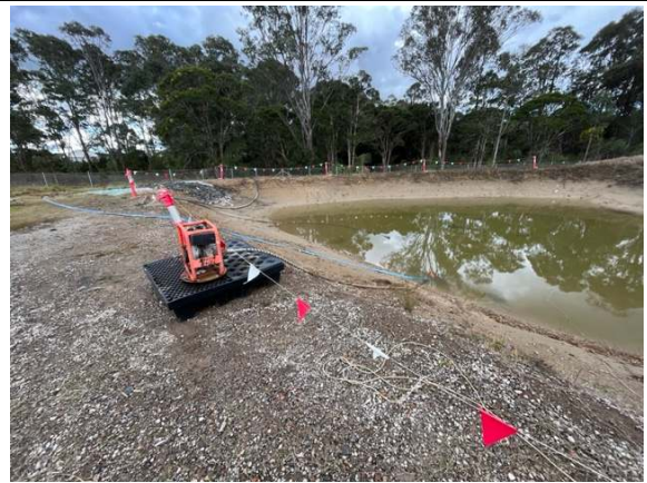
Photo 34: Sediment basin in place and in use for dust suppression
