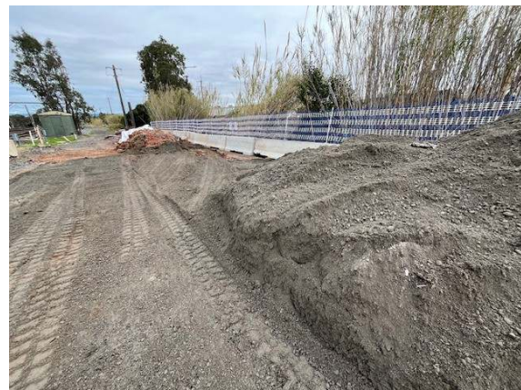
Photo 18: Stockpiling away from concrete barriers at Laydown 1. Stockpiles to be covered at end of shift.
