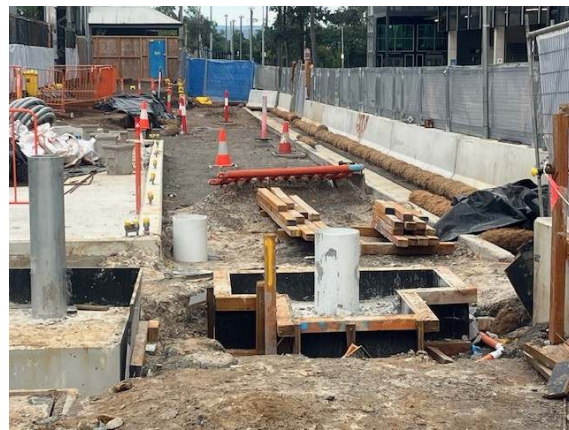
Photo 11: Coir logs in place along site boundary and isolated excavations.
