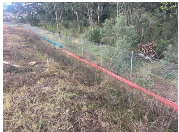
Photo 37: ERSed controls in place and no offsite impact observed on opposite side of earth bund
