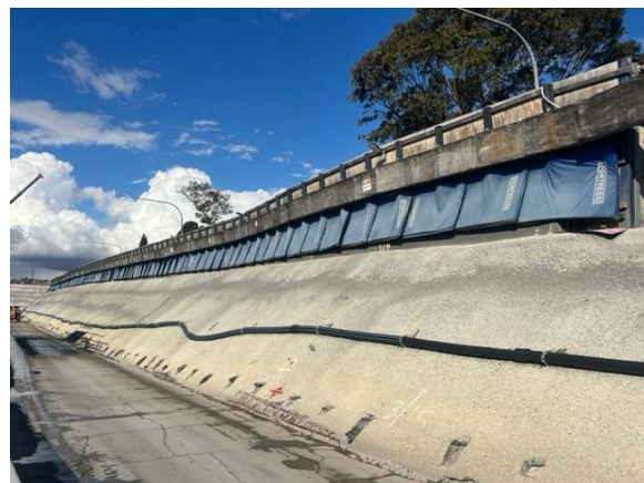
Photo 64: Noise blankets along street frontage – no gaps identified
