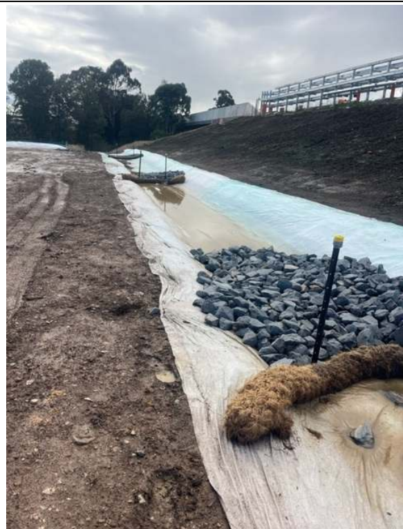
Photo 10: Swale to sediment basin with check dams and geofabric lining
