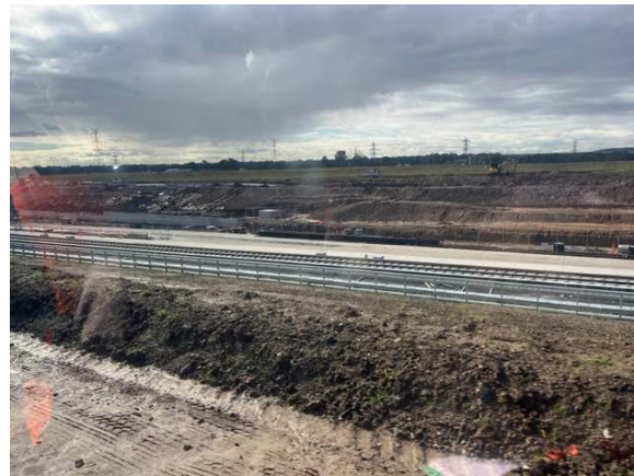
Photo 5: Rail & CSR works
