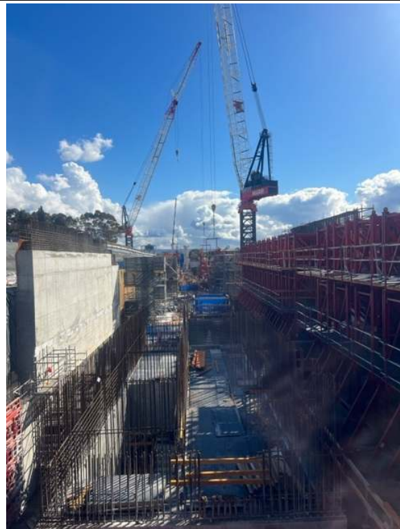
Photos 65 & 66: Station box. FRP works ongoing. Level B2 slab pour underway. Groundwater and rainwater seepage is pumped to the WTP. Working hours M-F 7am-6pm; Sat 8am-1pm
