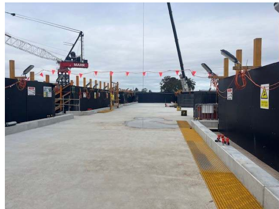
Photo 12: Works on the pedestrian bridge were ongoing with lighting pointed away from receivers.
