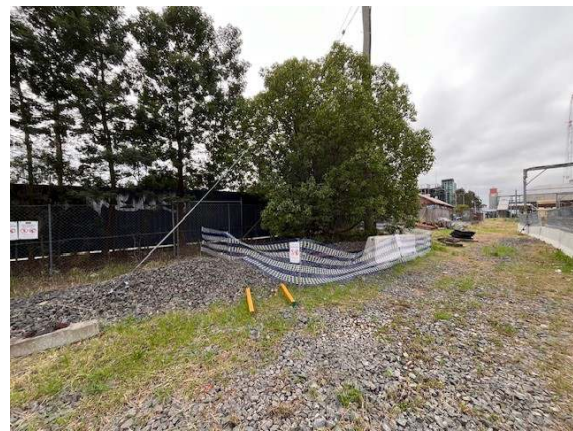
Photo 16: Tree protection was in place at Laydown 1.
