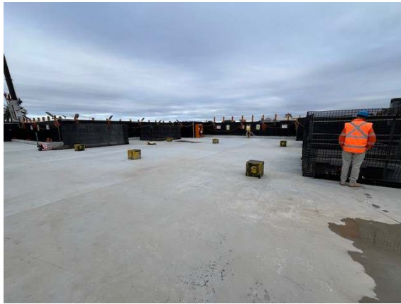
Photo 13: Works on the pedestrian bridge were ongoing – low environmental risk.
