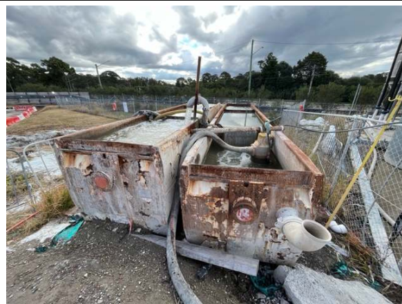
Photos 51 & 52: Water treatment plant operational – discharge to sewer via Trade Waste Agreement
