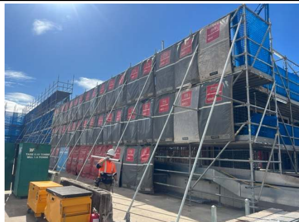
Photo 21 & 22: Concrete pour underway for operations building. Noise mats installed along resident-facing wall of building.
