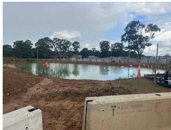
Photos 43 & 44: Sediment basin associated with licensed discharge point on other side of the road and Stand pipe for dust suppression
