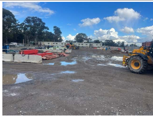
Photo 49: Site compound and laydown
