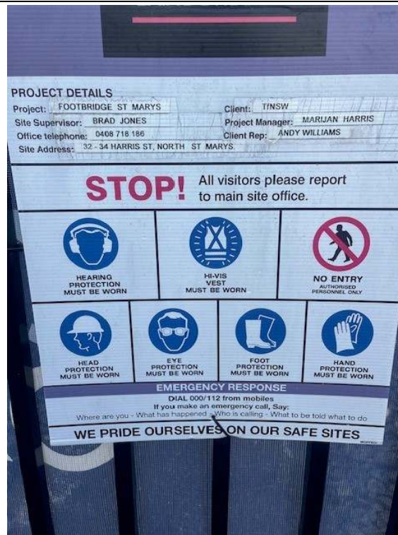
Photo 10: Signage in place at site entrance from Harris Street.
