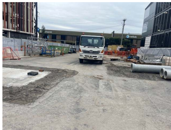
Photo 9: Material storage within the site compound on hardstand; good housekeeping and no tracking
