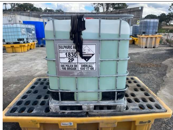
Photos 26-28: IBCs containing sulfuric acid were stored on bunds prior to transport offsite. The acid is no longer required after decommissioning of the WTP. Oil stored in IBC – to be identified and removed from site if not required
