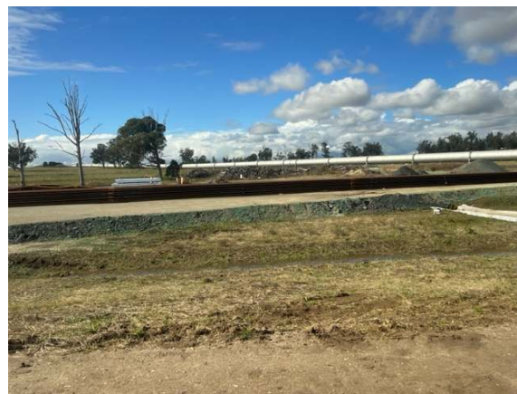
Photo 11: Linewide Portion 1C –Stockpile / laydown area near WaterNSW pipeline. Tree protection zones in place
