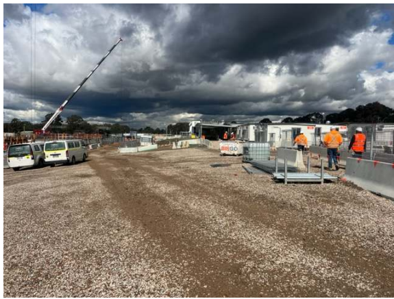
Photo 17: Site compound and stabilised internal haul road
