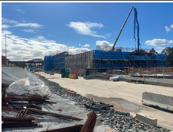
Photo 21 & 22: Concrete pour underway for operations building. Noise mats installed along resident-facing wall of building.
