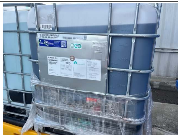
Photos 26-28: IBCs containing sulfuric acid were stored on bunds prior to transport offsite. The acid is no longer required after decommissioning of the WTP. Oil stored in IBC – to be identified and removed from site if not required
