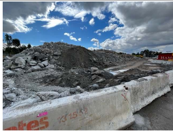
Photo 29: Concrete stockpiled for future crushing for internal road construction during standard construction hours
