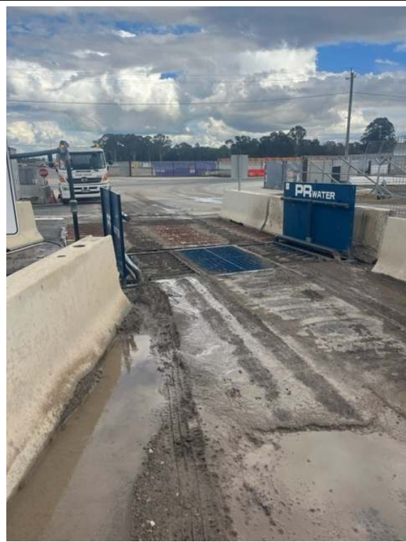
Photos 45 & 46: Wheel wash and signage at front gate
