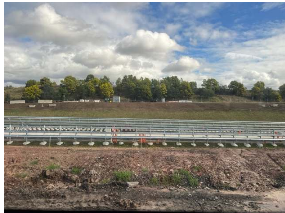
Photo 12: CSR works complete and backfill and stabilisation scheduled to commence
