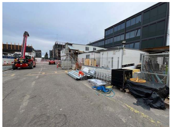
Photo 4: Site compound on hardstand and materials storage.
