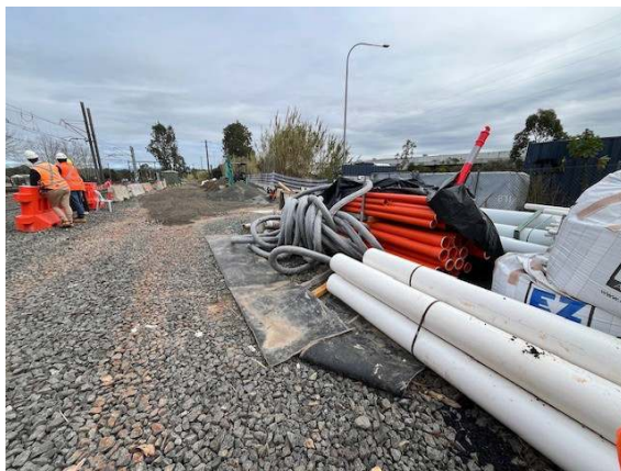
Photo 17: Inert materials storage and stabilised internal access at Laydown 1.
