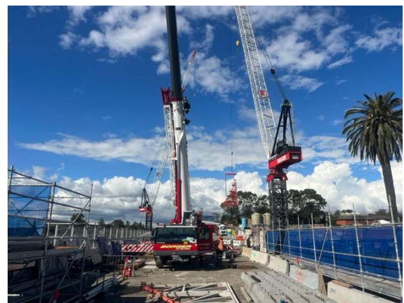
Photo 63: Diesel Cranes operational for lifts into station box. A 250m3 slab pour was underway
