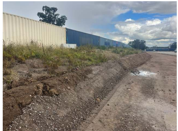
Photo 38: Noise wall in place and weed management ongoing
