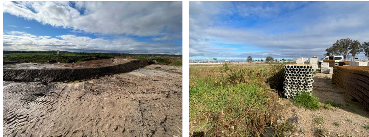
Photos 1 & 2: Concrete washout bay and laydown. Weeds had been sprayed within the laydown. BND has been engaged to conduct weed management and maintenance of landscaped areas across the project.
