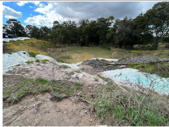
Photo 30: Sediment basin in place and in use for dust suppression
