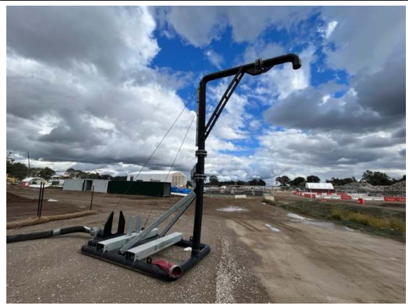
Photos 31 & 32: Sediment basin – water reused for dust suppression or pumped to Claremont Meadows WTP. stand pipe for dust suppression
