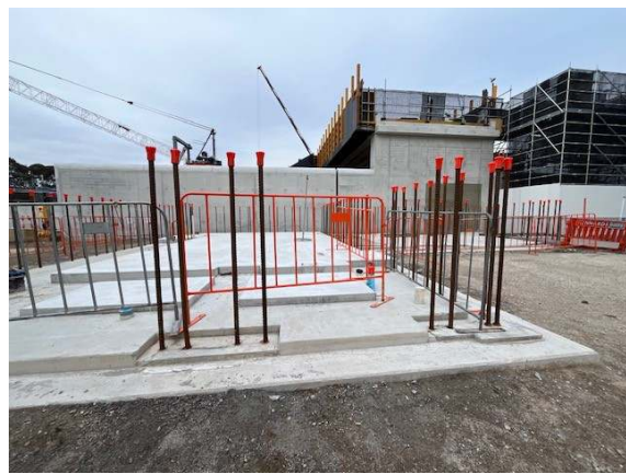
Photo 8: Base slab poured for Sydney Trains building.
