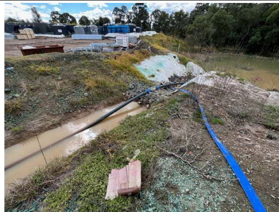
Photos 31 & 32: Sediment basin – water reused for dust suppression or pumped to Claremont Meadows WTP. stand pipe for dust suppression
