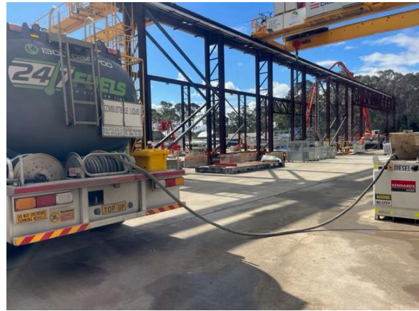
Photo 18: Refuelling of diesel cell underway. Spill kit in place and operator observing
