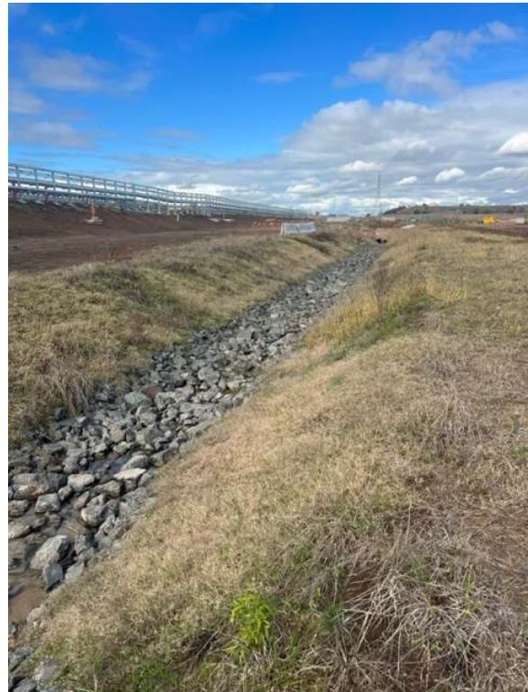
Photo 8: Swale to sediment basin
