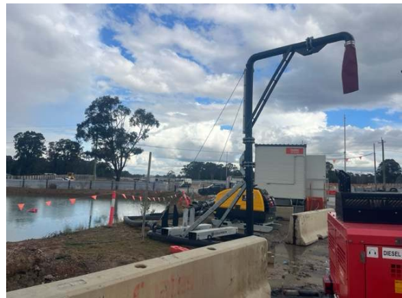
Photos 43 & 44: Sediment basin associated with licensed discharge point on other side of the road and Stand pipe for dust suppression
