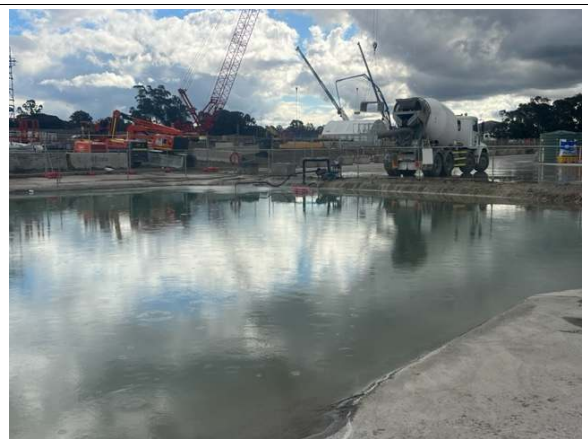
Photo 42: Water diverted to holding basin from concrete batching plant. Water is reused in the
