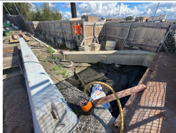
Photo 62: Rainwater accumulating in low points was pumped to the WTP
