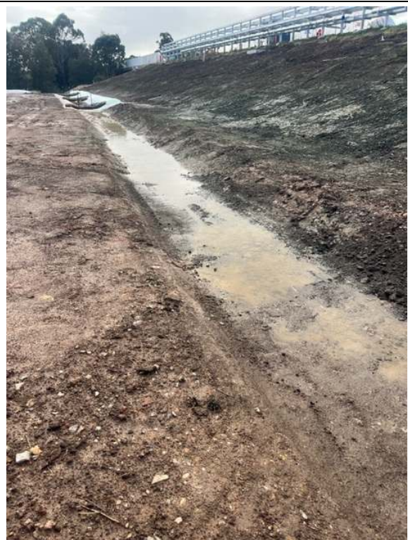
Photo 9: Discharge swale from sediment basin line with polymer
