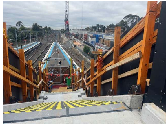
Photo 14: Access to platforms and view of adjacent SSTOM St Marys station site.
