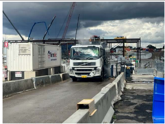
Photo 25: The wheel wash was in use and effective
