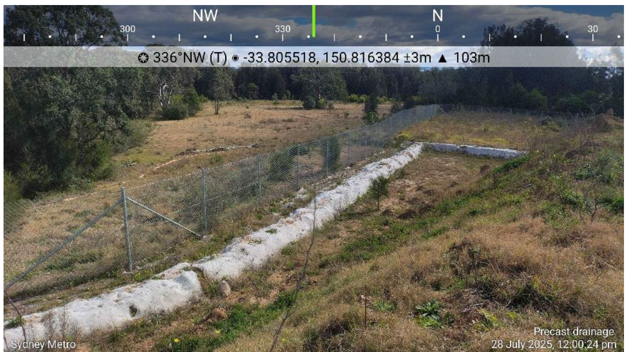
Figure 6-2 Area north north-west adjacent to the proposal area
