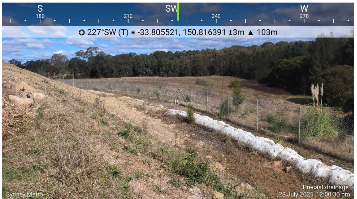
Figure 6-4 Area west of the existing sediment basin, where the discharge route would be constructed
