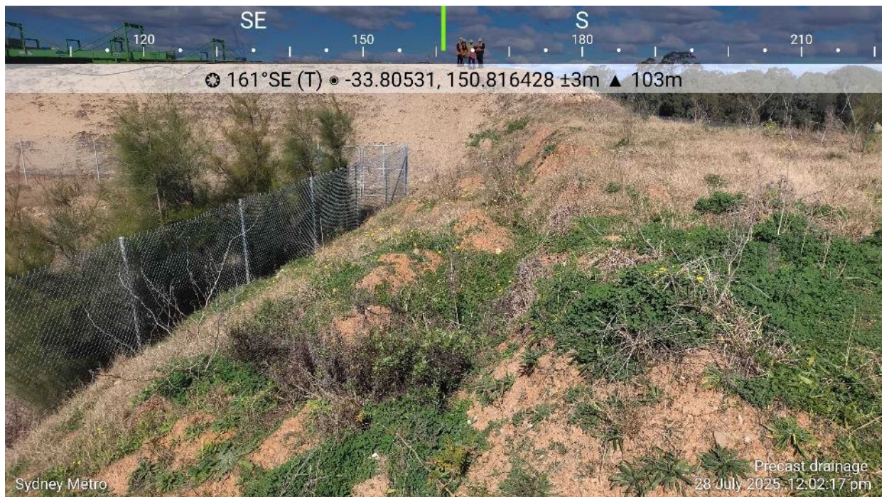
Figure 6-5 Area west of the existing basin looking south to where the discharge route would be constructed
