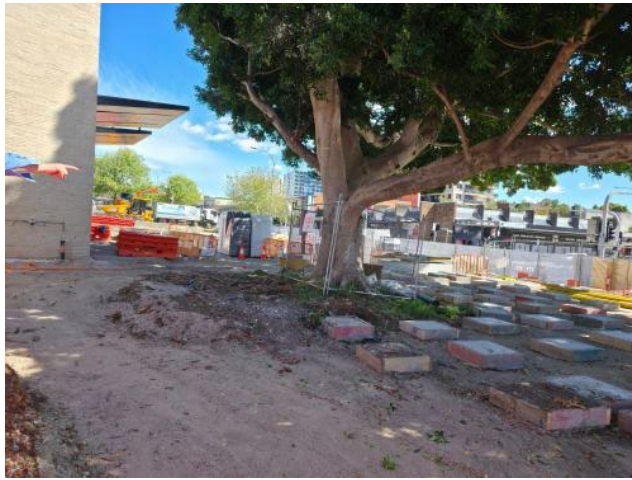
Figure 1 – Bankstown - Preparations works for concrete poured footings for timber deck (around fig tree) and stairs ongoing.
