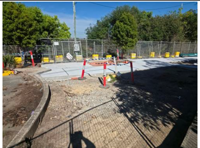
Figure 4 – Bedford Crescent, Dulwich Hill - Landscaping, footpath and tiling works in progress.
