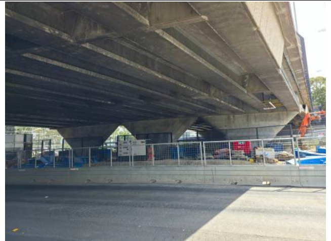
Figure 2 – Stacey St, Bankstown – South Terrace - Bridge Strengthening works completed at this site. Martinus reported that plant/equipment was in the process of being demobilised.
