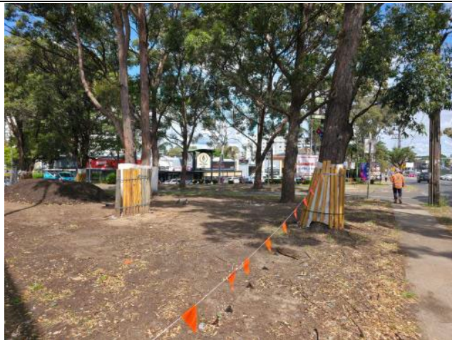
Figure 3 – South Terrace Minor Ancillary Facility – Demobilisation ongoing post-completion of works in this area. Topsoil placement and landscaping works ongoing.
