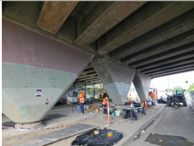
Figure 1 – Stacey St, Bankstown – Bridge strengthening works ongoing.
