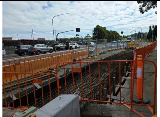
Figure 4 – Stacey St – Stage 2 – Footpath works including form, reo and pour (FRP) ongoing.
