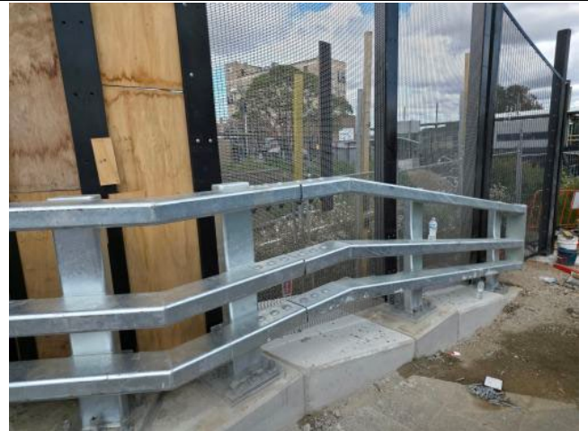
Figure 6 - Haldon St, Lakemba - Barrier installation nearing completion at all location near Haldon St.
