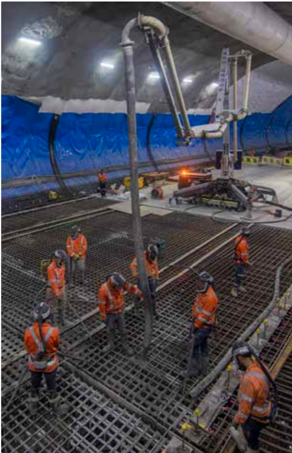
Concreting and waterproofing the crossover cavern.
