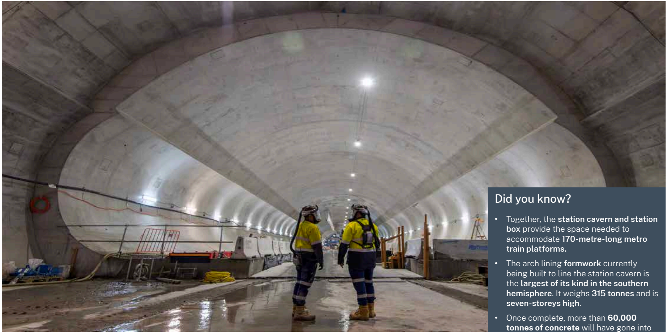
Waterproofing and lining works complete inside the rail crossover cavern.
