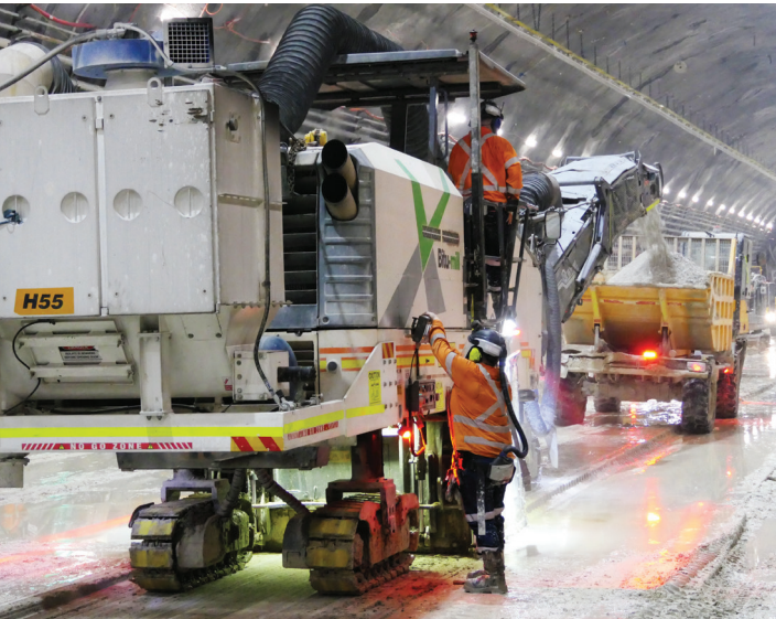
A profiler is a machine used to excavate the cavern invert by slowly grinding away the surface of the rock.
