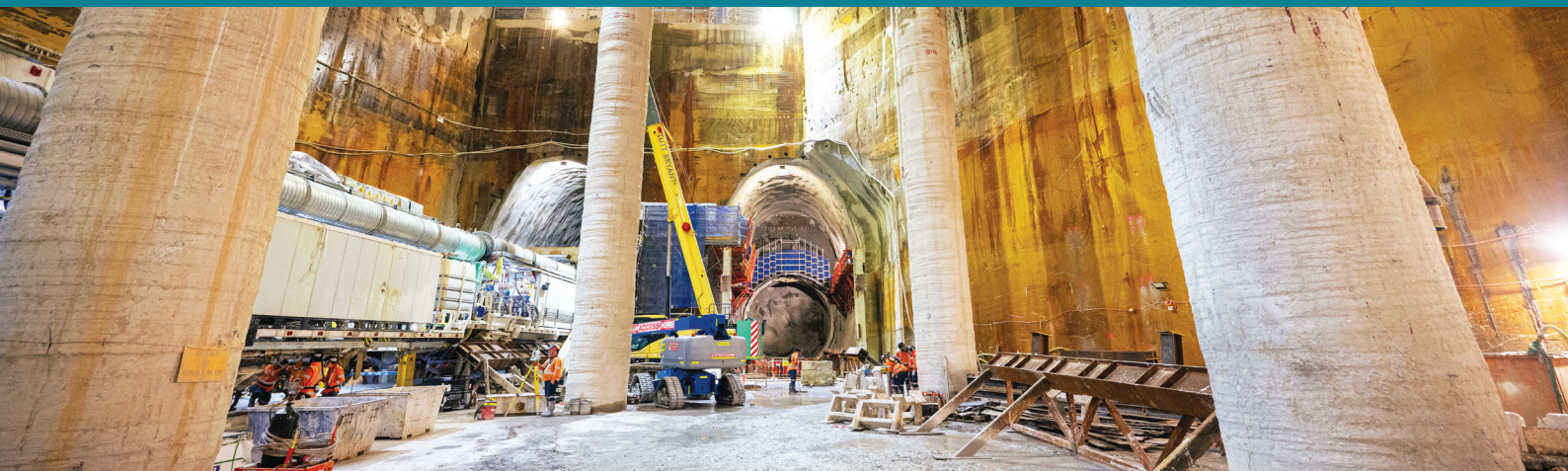
TBM Ruby traverses (passes through) the base of the 33-metre deep shaft at Pymont East.
