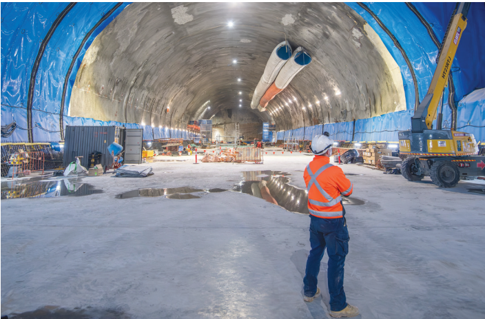
An example of a completed invert pour.
