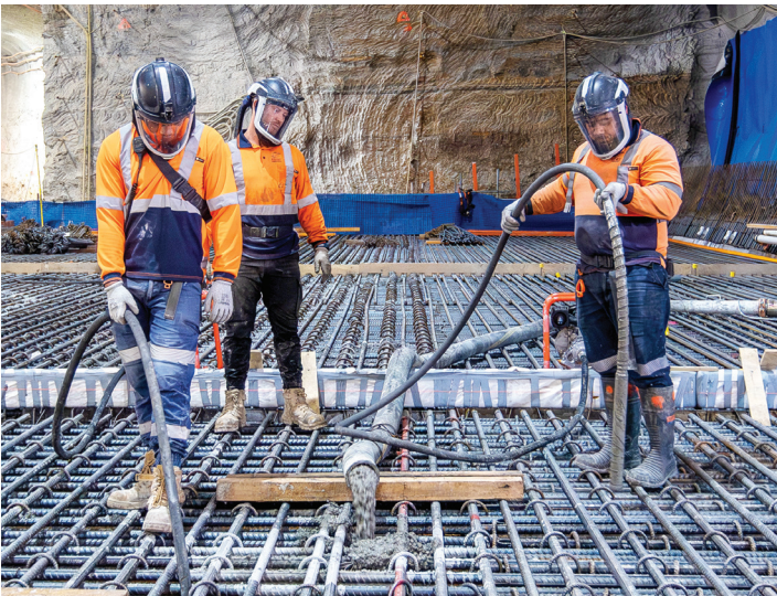
The concrete pours from Union Street will be used to line the Pyrmont cavern and adits.
