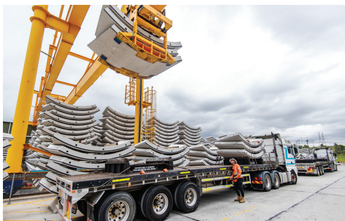
Concrete segments will be brought to Pyrmont via truck and lowered into the Pyrmont cavern via a crane inside the acoustic shed.
