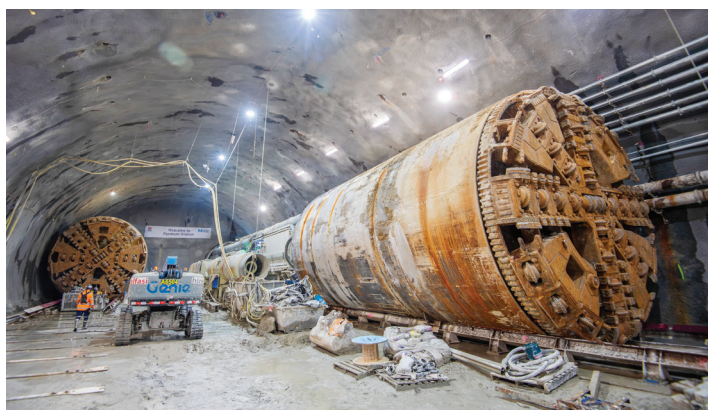
TBM Ruby, pictured right, was the first mega borer to break through into the Pyrmont cavern.
