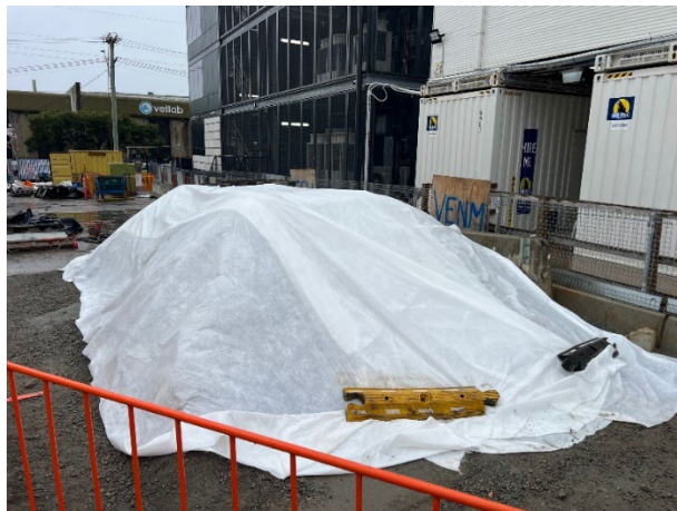
Compound: The stockpile of DGB was covered in geofabric before the commencement of the rain, this is good practise.
