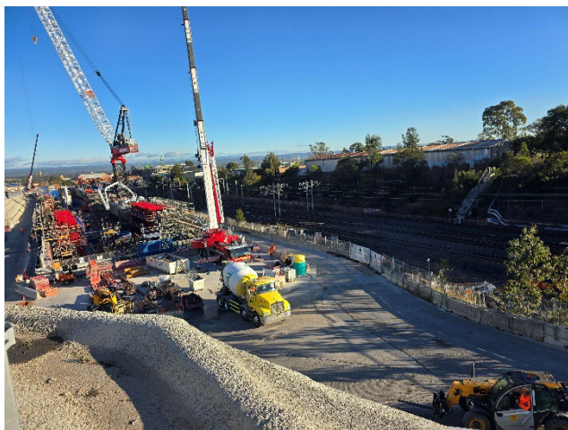
STM – Concrete pout on eastern end of box – washout was observed into trays, and spill controls in place.
