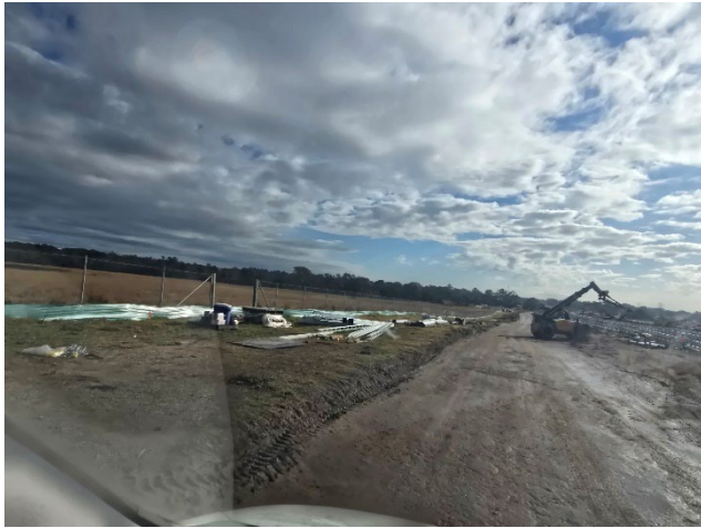
Lansdowne Rd to Patons Ln – Laydown of GST on vegetated stabilised areas – raised with PLM that stabilised areas should be maintained where possible and ECMs updated to show approved laydown areas as ancillary facilities.
