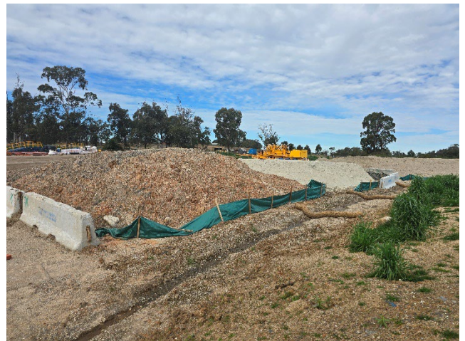
BSF – Reinstatement of sediment fence was required post rainfall.
