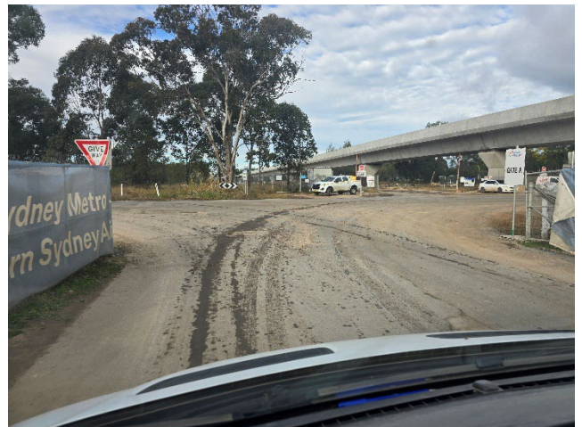
SMF – Minor tracking onto Patons Lane – rumble grids installed and street sweeper operating.
