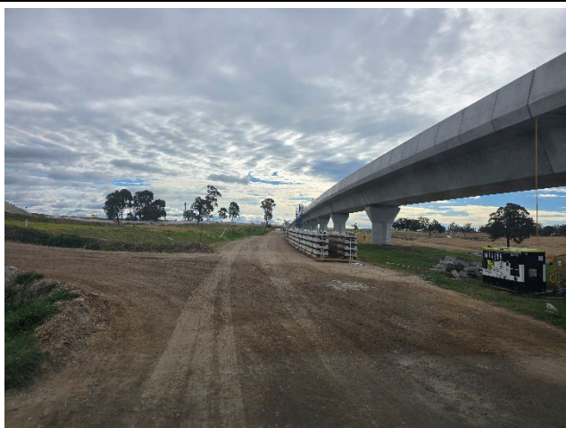
Luddenham to M12 – Sleeper deliveries on stabilised haul road (good practice).
