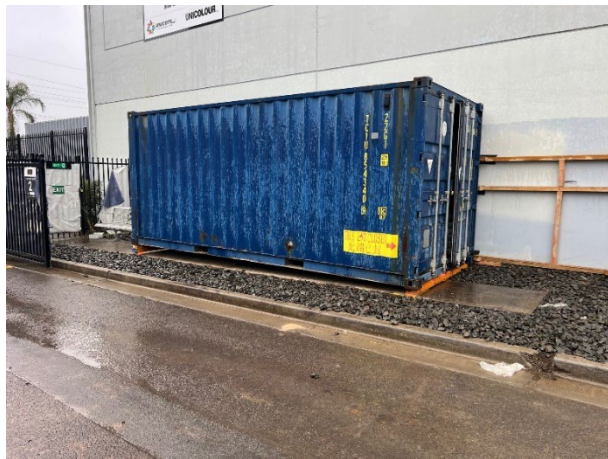
Compound: Ballast has been placed to minimise ground disturbance while area is used for storage.
