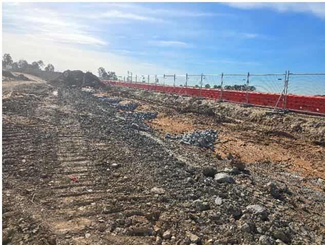
BRD – Drainage line with rock checks and importing shale for backfilling.
