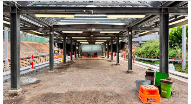
Figure 10 - Bankstown - Sydney Trains side platforms – asphalt removal complete.
