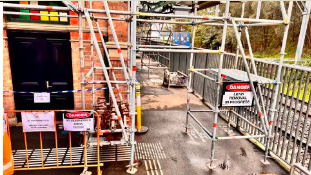
Figure 1 – Canterbury Station – Platform works including lead removal, asphalt removal and roofing ongoing.
