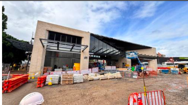
Figure 5 – Bankstown Station – Steel works completed, internal fitout, brick and block works ongoing.
