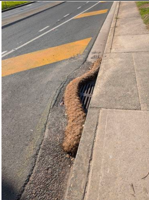
Figure 1 – Stacey St, Bankstown – Erosion and sediment controls in place around stormwater drains.
