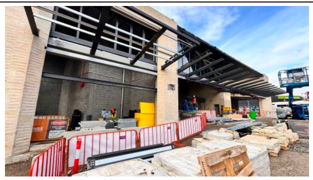
Figure 4 – Bankstown Station - Station Works: Mechanical, electrical and plumbing works ongoing including LV rough in, storm water pipes work.
