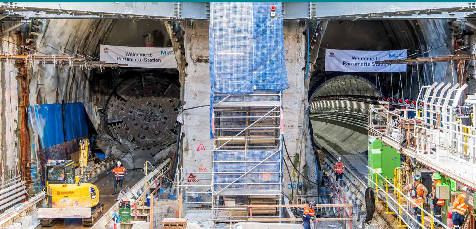
Tunnel boring machine (TBM) Dorothy at the entrance to the station box, with TBM Betty already on her way to Westmead
