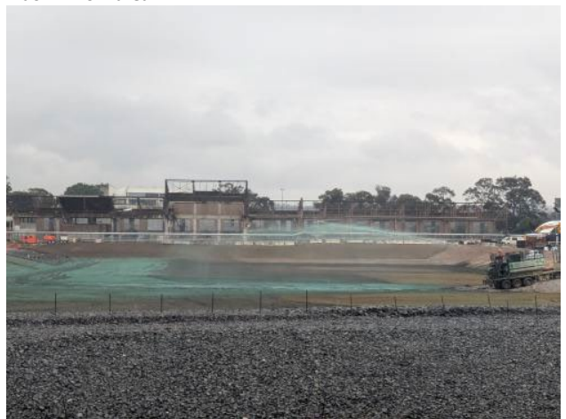
Figure 2.14 – Clyde MSF Site: Flood basin - hydromulching in progress.
