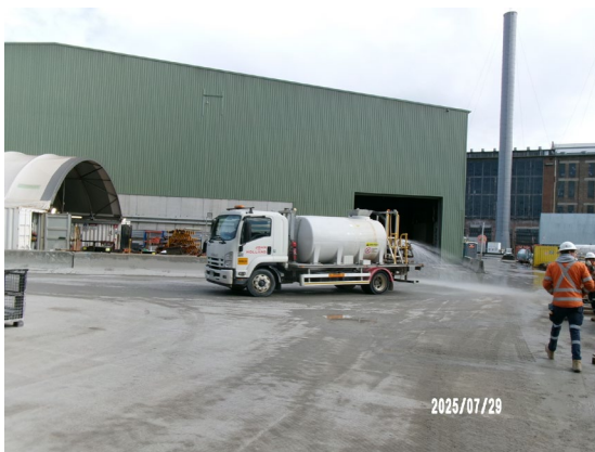
Figure 3.9 The Bays: Use of water cart for dust suppression.
