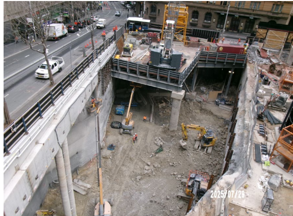
Figure 3.2 Hunter Street East: Excavation adjacent Hunter Street and load out of spoil from the steel deck.
