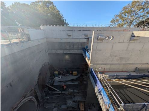
Figure 2.9 – Clyde Dive Site: Lining Erection Machine (LEM) re-launched. GLC reports ring building ongoing.
