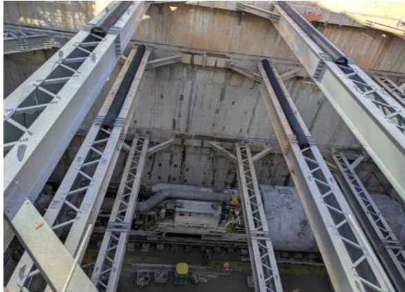
Figure 2.1- Parramatta Site: TBM 1 traversing through station box.
