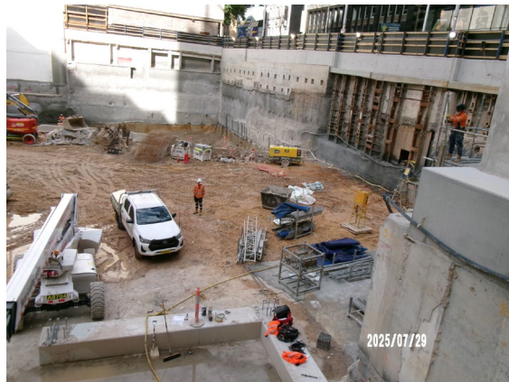
Figure 3.4 Hunter Street West: Ongoing excavation; wall support and steel deck footings.
