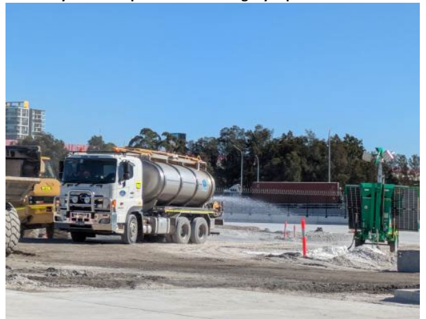
Figure 2.12 – Clyde MSF Site: Water cart mobilised and wetting down work area.
