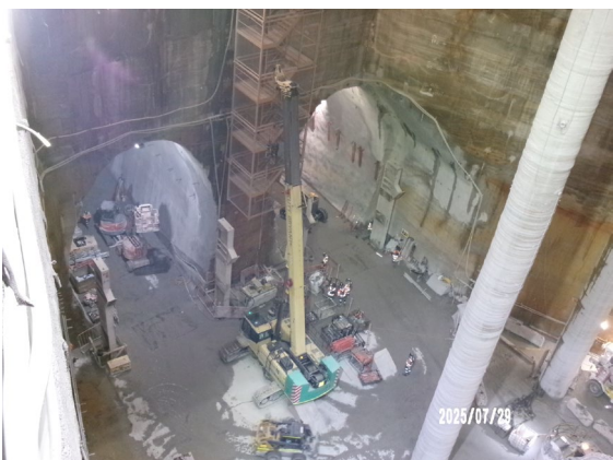
Figure 3.5 Pyrmont East: Shaft excavation completed. Works in the nozzles to prepare for TBM re-launch.
