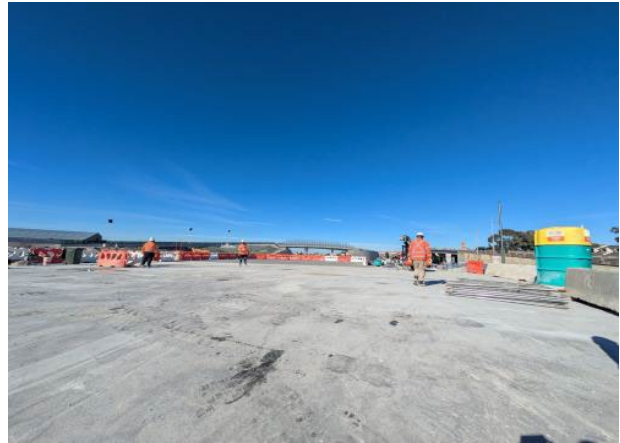
Figure 2.10 – Clyde Dive Site: Final formation around HV protection and utility slabs completed and blinding layer poured.
