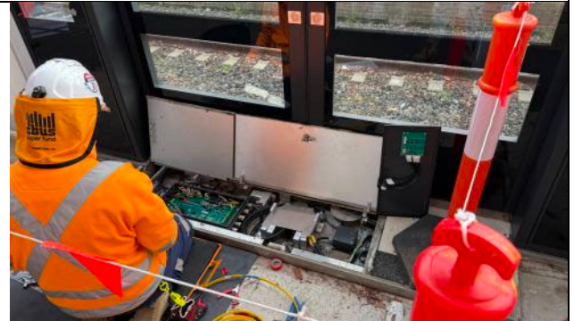
Figure 4 – Marrickville Station – Electrical activities associated with platform screen doors and mechanical gap fillers underway.
