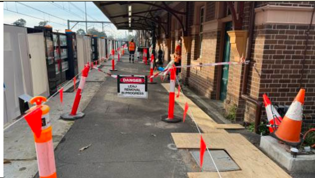
Figure 1 – Marrickville Station – Lead removal in progress inside the station buildings. Lead removal related air quality sampling was being undertaken at the time of inspection.
