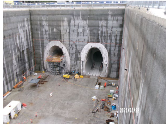
Figure 1.8 Remedial works in the nozzles (SOP).
