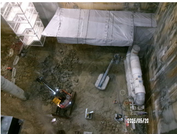
Figure 3.7 Pyrmont West: Preparation to excavate an adit with the road header.
