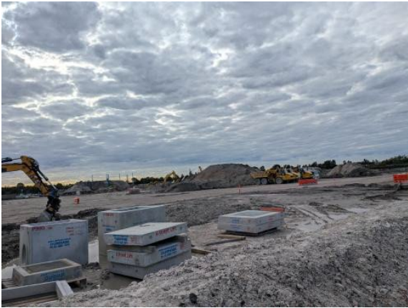
Figure 2.11 – Clyde MSF Site: Stormwater drainage works underway.
