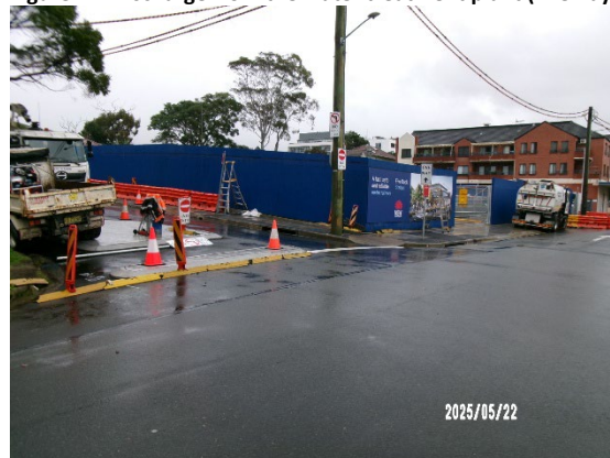
Figure 1.4 Hoarding installed around the east site. Reinstatement of footpaths (Five Dock).
