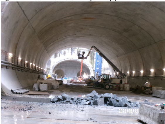
Figure 1.3. Removal of blinding concrete in the eastern shaft (Five Dock).
