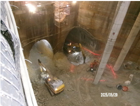
Figure 3.5 Pyrmont East: Nozzle excavation by road header completed with ongoing excavation by rock hammer.
