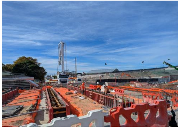
Figure 2.12 – Clyde Dive Site: HV protection slab - FRP works ongoing.
