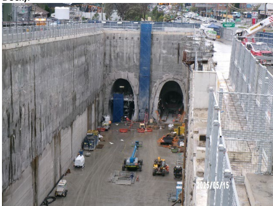
Figure 1.5 Remedial works ongoing in the nozzles (Burwood North).
