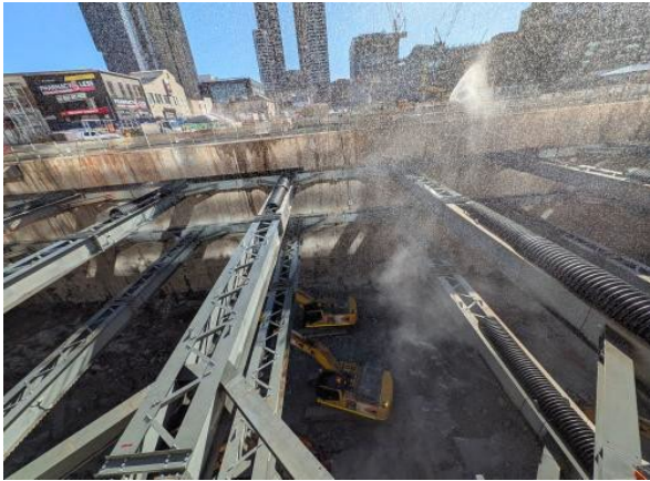
Figure 2.1- Parramatta Site: Dust suppression measures in place for box excavation.
