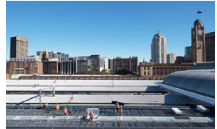
Solar panels are being installed as part of Sydney Metro's major upgrade of Central Station.
