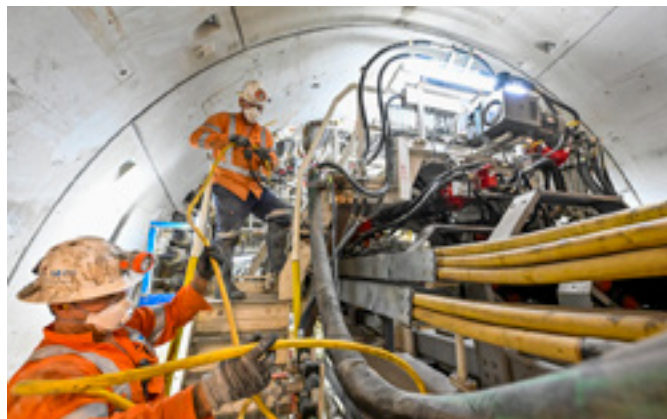
Installation of tunnel segments.
