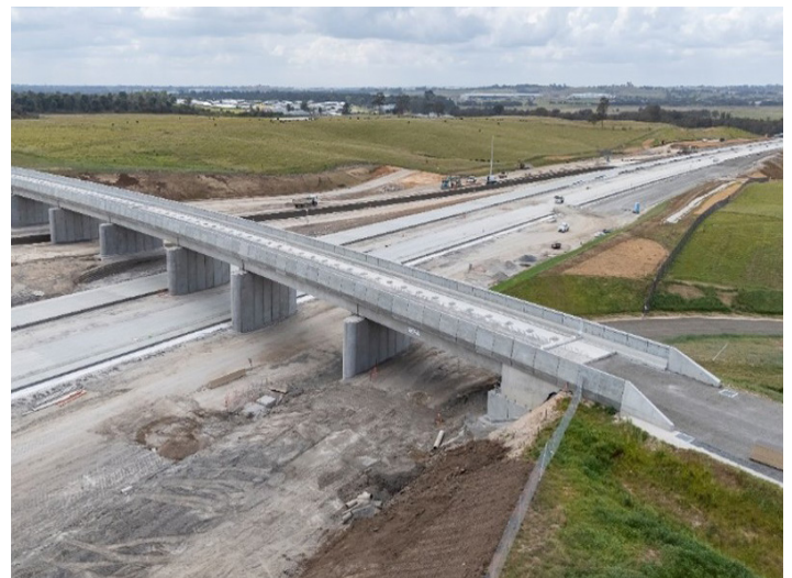
A view of the 190-metre rail bridge constructed over the new M12 Motorway project.
