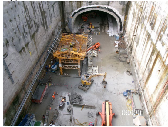
Figure 1.4 Removal of the lining formwork; general activities in the western shaft (Five Dock).
