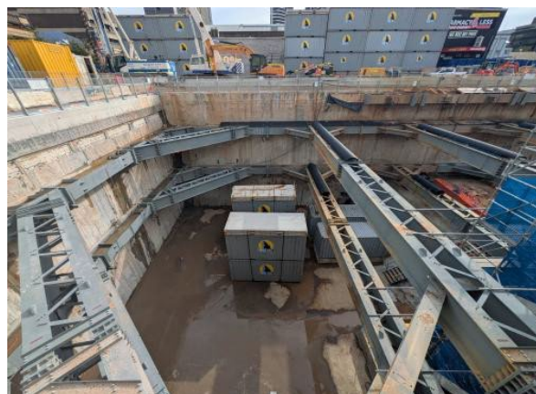
Figure 2.2- Parramatta Site: Staged container wall removal and piling; with temporary container storage in Western Station Box.
