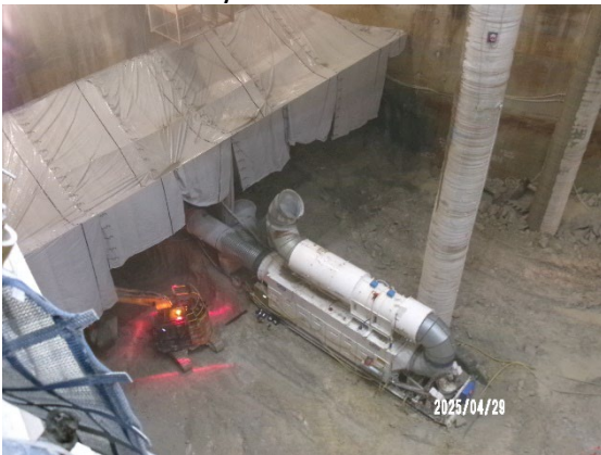
Figure 3.5 Pyrmont East: Nozzle excavation by road header with new scrubber unit operating.
