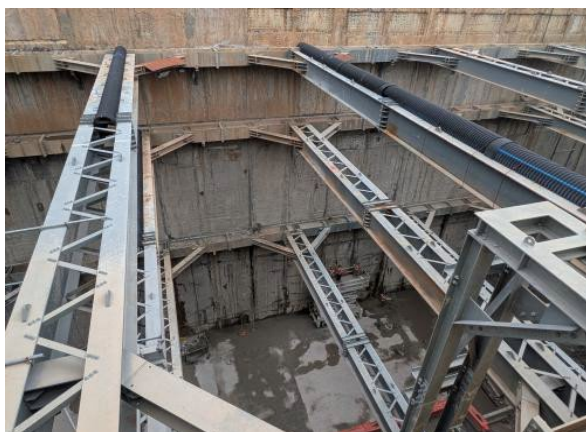
Figure 2.1- Parramatta Site: D-Wall rectification works in Eastern Station Box.
