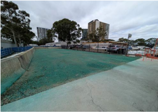
Figure 2.9 – SOP Site: Polymer sprayed on previous site shed area. ERSED controls remain on batter.
