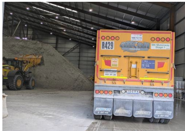
Figure 2.14 – Rosehill Site: Spoil storage and truck loadout within shed.
