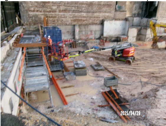
Figure 3.3 Hunter St West: Construction of the capping beam along Hunter Street boundary.
