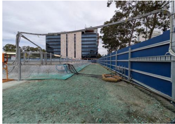
Figure 2.10 - SOP Site: Sediment controls remain; with polymer sprayed on area adjacent to the Station Box.
