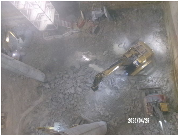
Figure 3.7 Pyrmont West: Excavation of the permanent shaft using multiple rock hammers.
