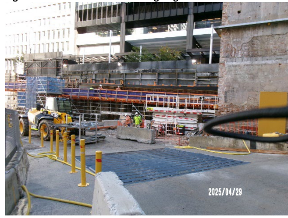
Figure 3.4 Hunter Street West: New access concrete access with rumble grid and capping beam in background.
