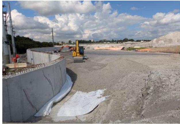
Figure 2.16 – Clyde MSF Site: Section 6 – GLC reports piling works for ground improvement completed in area and backfilling progressing.
