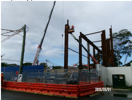
Figure 1.3. Removal of the acoustic shed frame (Five Dock East).
