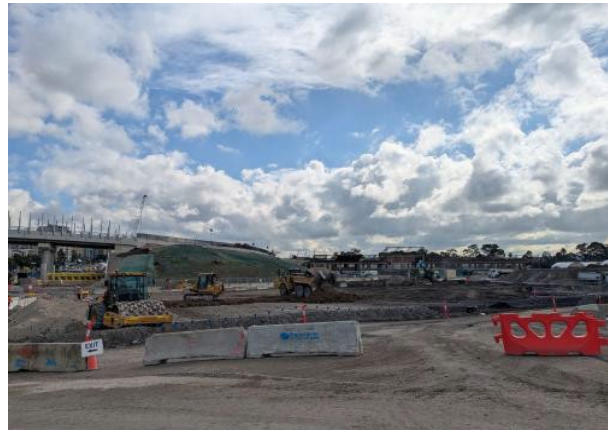
Figure 2.12 – Clyde MSF Site: Backfilling and levelling of previous MSF West shed area continuing.
