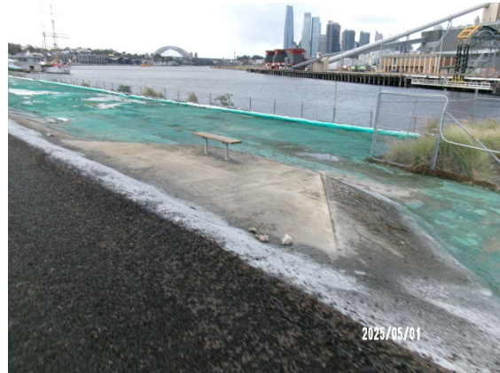
Figure 1.2 Polymer placed on soil areas adjacent the harbour (The Bays).
