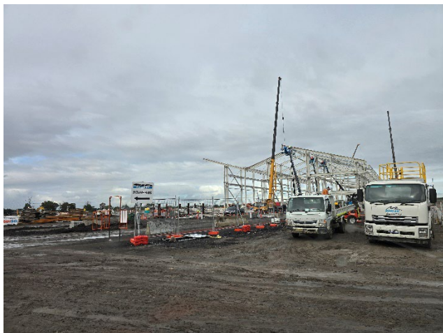
SMF – Building structural steel installation commenced.
