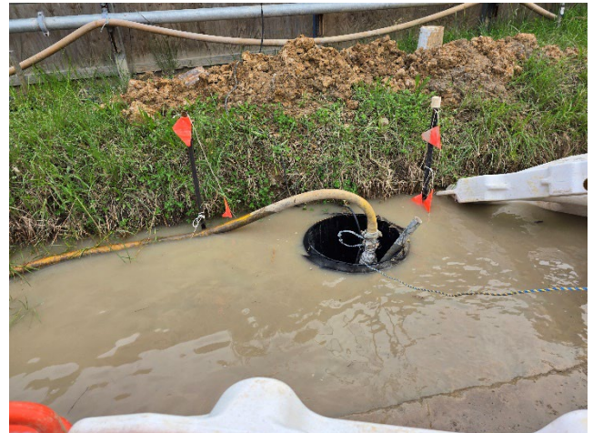
CMSF – Sump installed adjacent to shaft pad.
