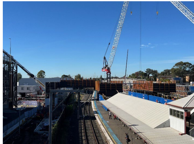
Station overpass: Works over the platforms are enclosed in hoarding.
