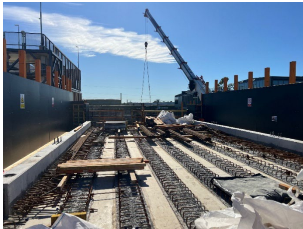
Platform 1/2: Beams have been lifted into place from the compound to platform 1/2.
