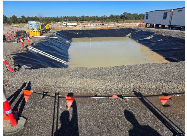
BRD – New basin to be connected to surface water drainage.
