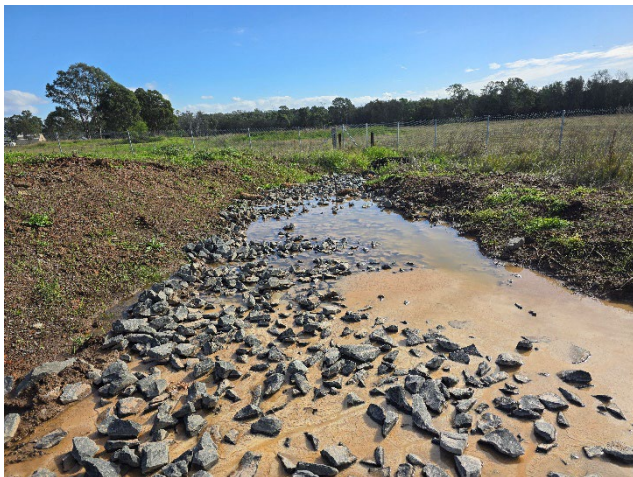
BSF – Flock blocks dropping out sediment in laydown controls.
