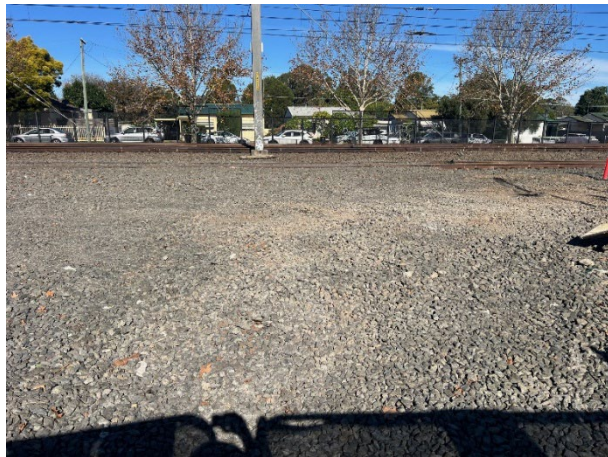
MAF1: Additional ballast has been added to the entry / exit point.
