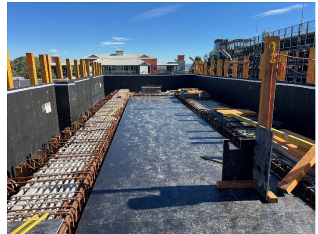
Platform 1/2: The deck has been prepared for concrete pours over the coming weeks.
