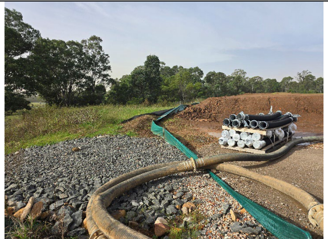
OHE – A water hose had been placed on the sediment fence. PLM immediately arranged for this to be removed and discussed options for better ESC measures to permit pumping activities for water carts.
