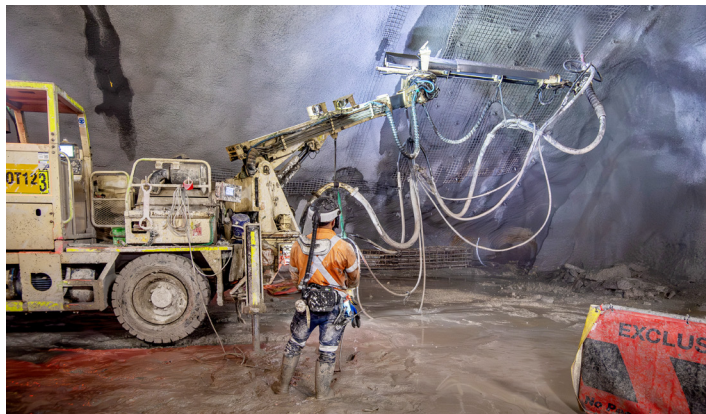
A concrete mixture (shotcrete) is sprayed to the wall of the cavern to provide support.
