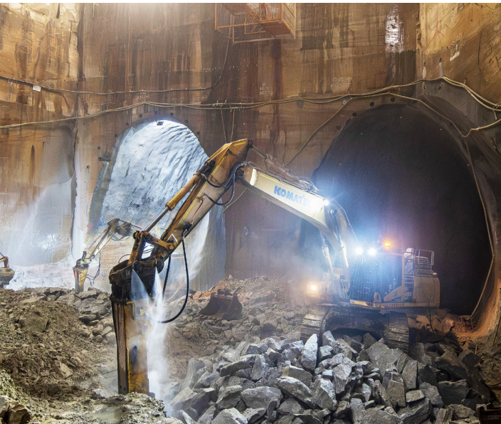
Pymont East shaft excavation.
