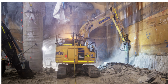
A rock hammer being used during shaft excavation to break up ground material.
