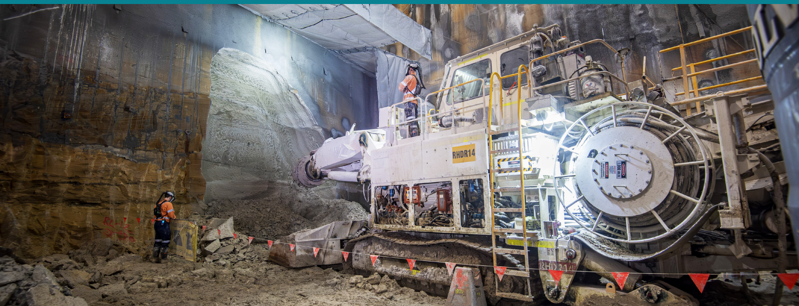
Four roadheaders are working simultaneously underground to excavate the Pyrmont station cavern and tunnels.
