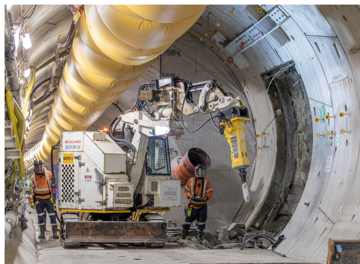
Cross passage excavation in the TBM Jessie tunnel.
