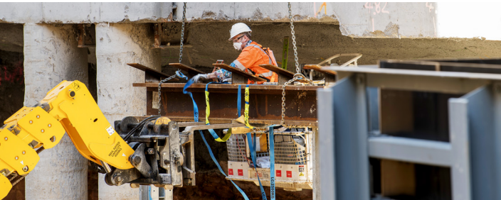
A beam is installed beneath the Hunter Street footpath as part of the eastern shaft niche excavation.
