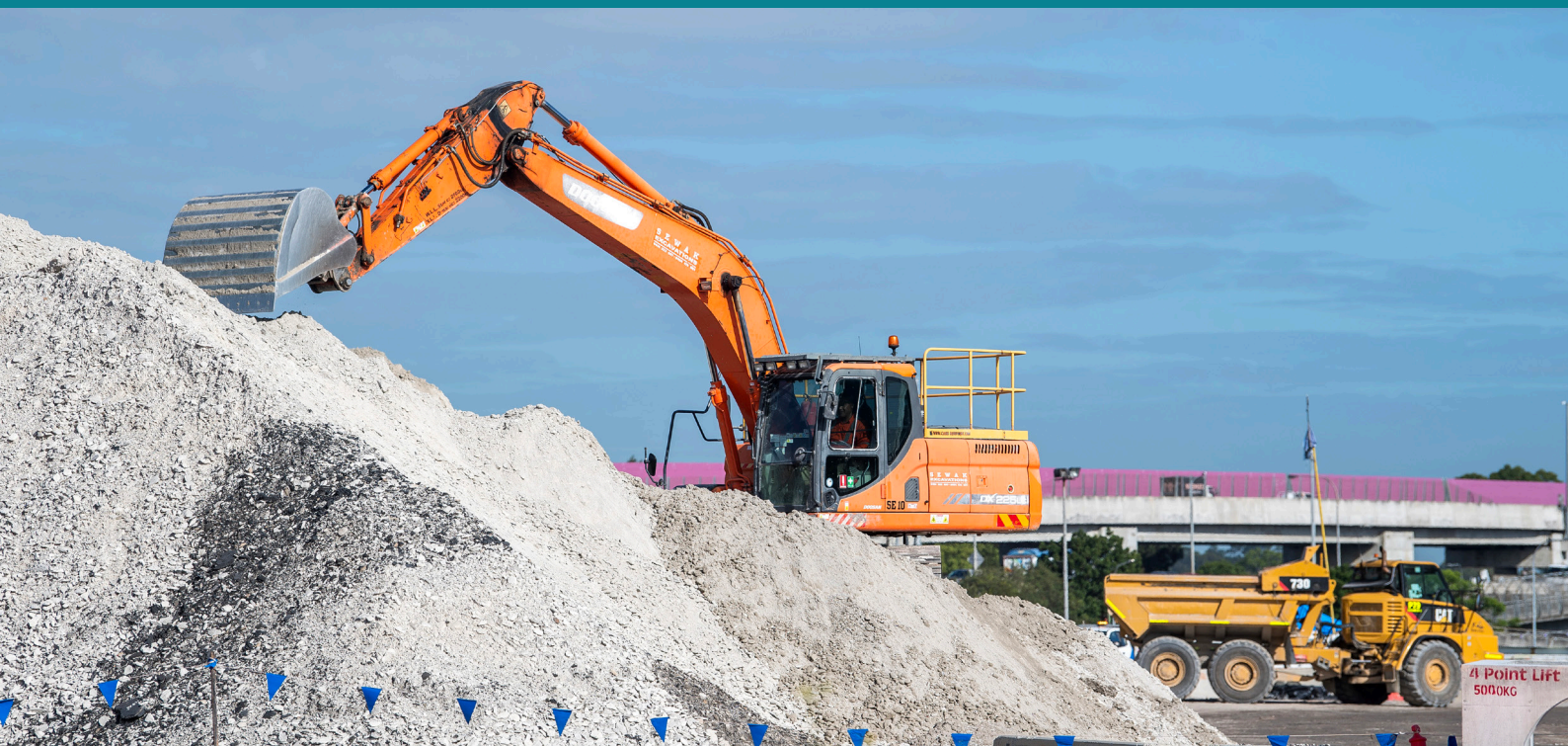
Hawkesbury sandstone excavated during tunnelling, being reused at Clyde stabling and maintenance facility
