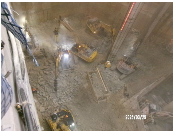
Figure 3.5 Pyrmont East: Shaft excavation by rock hammers.
