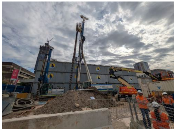
Figure 2.3 – Parramatta Site: Staged container wall removal, piling and stockpiling works.
