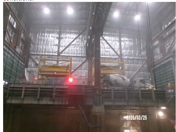
Figure 3.6 Pyrmont East: Use of kibbles for spoil load out.
