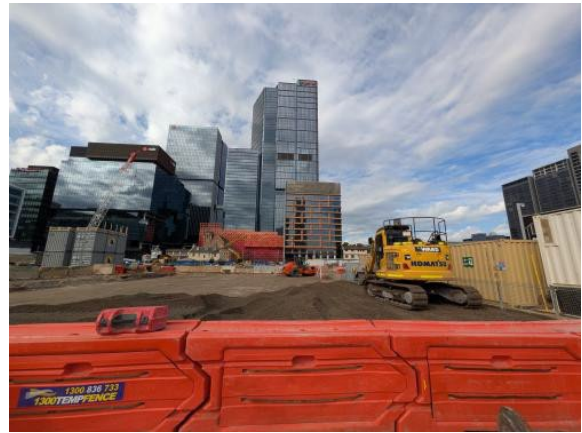
Figure 2.2- Parramatta Site: Zone 8a backfilling and levelling works.
