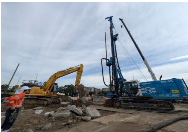
Figure 2.11 – Clyde Dive Site: Piling work for HV Protection Slab works.
