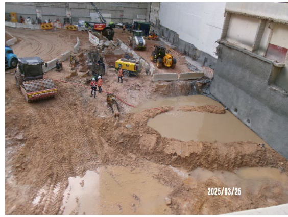
Figure 3.4 Hunter Street West: Water management in wet conditions.
