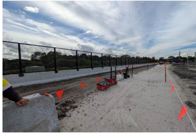
Figure 2.14 – Clyde MSF Site: Section 7 (Slip form area) – Screen and barrier installation works.
