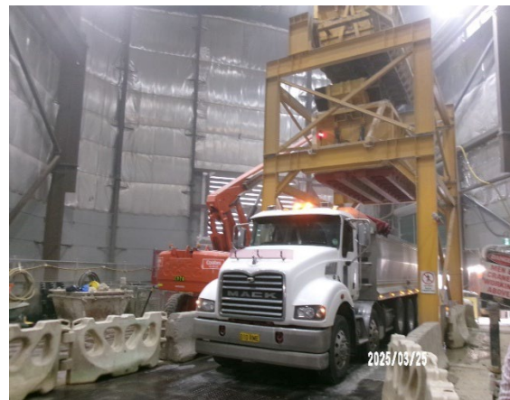
Figure 3.8 Pyrmont West: Use of kibble to load trucks.
