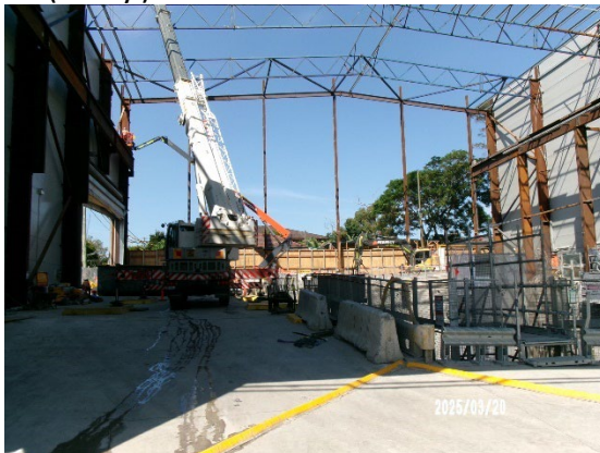
Figure 1.3. Removal of the acoustic shed (Five Dock East).
