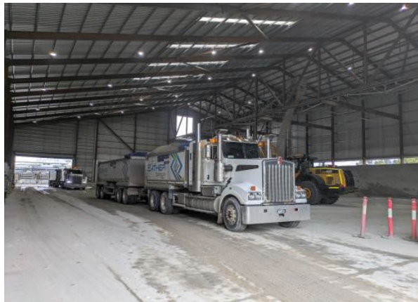
Figure 2.9 – Rosehill Site: Spoil load-out within shed at Rosehill.
