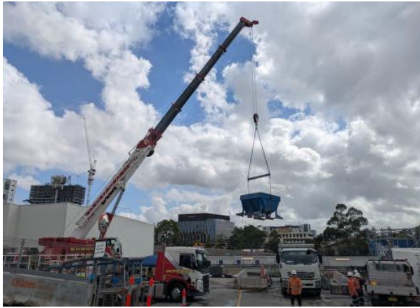
Figure 2.7– Westmead Site: Spoil load out via crane and kibble.
