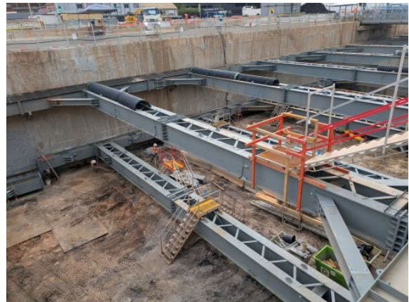
Figure 2.4 – Parramatta Site: Installation of struts and walers – Central Station Box.
