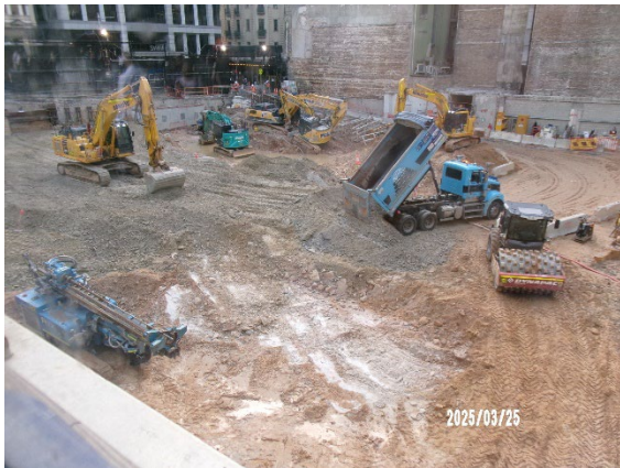
Figure 3.3 Hunter St West: Construction of piling pad.
