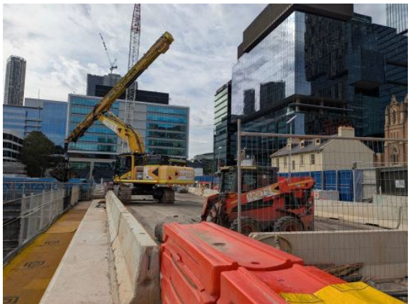
Figure 2.5 –Parramatta Site: Spoil load out from Central Station Box.
