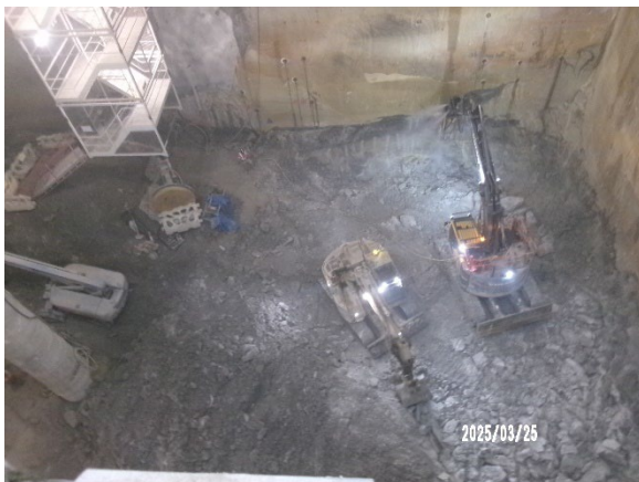
Figure 3.7 Pyrmont West: Excavation of the permanent shaft.
