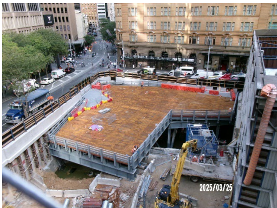
Figure 3.1 Hunter Street East: Construction of the steel deck completed by the end of the month.
