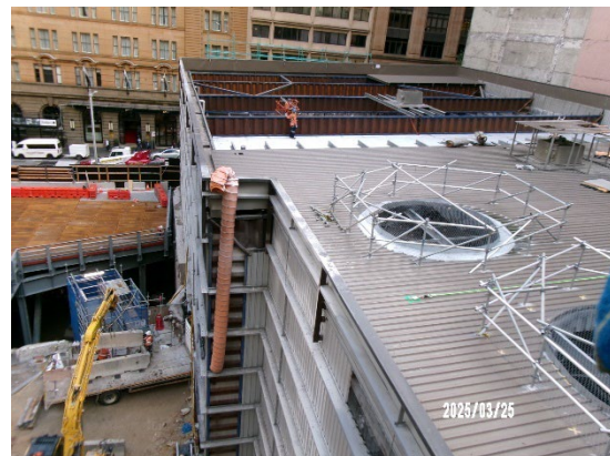
Figure 3.2 Hunter Street East: Removal of the shed roof.
