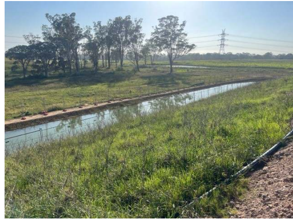
Photo 1 & 2: Temporary sediment basin in place. Water from this basin is pumped to the main sediment basin as required prior to testing and reuse on site for dust suppression.
