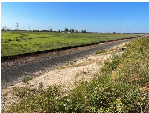
Photos 5 & 6: Swale along the eastern site boundary with rock check dams and sediment fencing at an identified low point.
