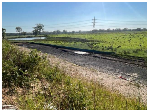
Photos 5 & 6: Swale along the eastern site boundary with rock check dams and sediment fencing at an identified low point.
