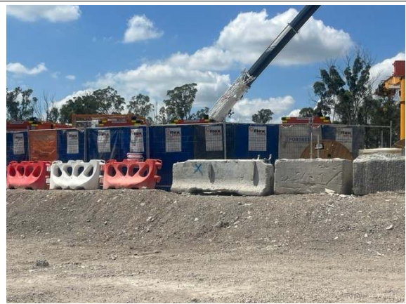
Photo 27: Noise blankets were installed on generators but had been installed on the wrong (non-resident) side, as identified by the PLM Environmental Advisor. PLM to rectify under their own system.
