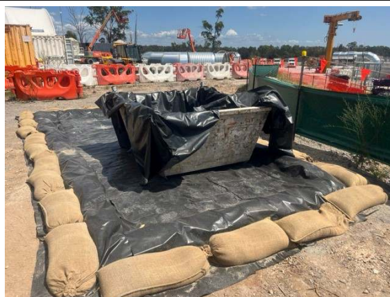
Photo 21: A concrete washout had been established with controls in place
