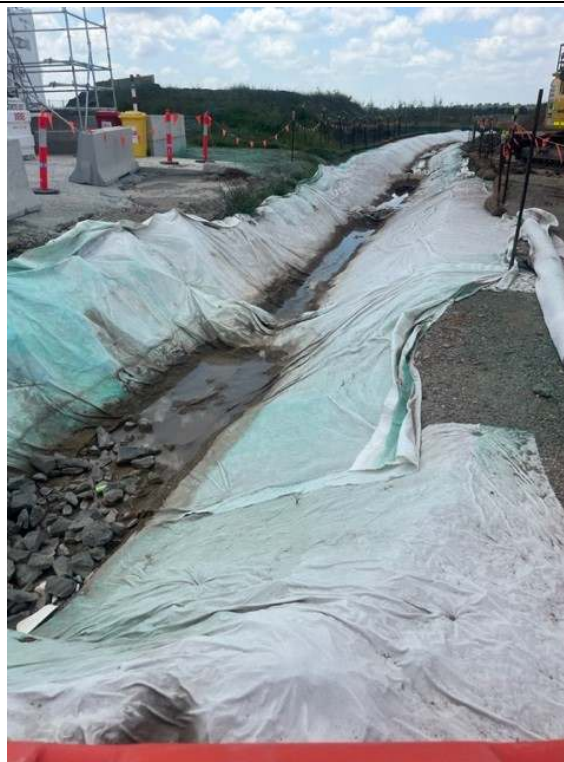
Photo 36: A clean water diversion was in place and controlled with geofabric and rock checks, as required by the ESCP
