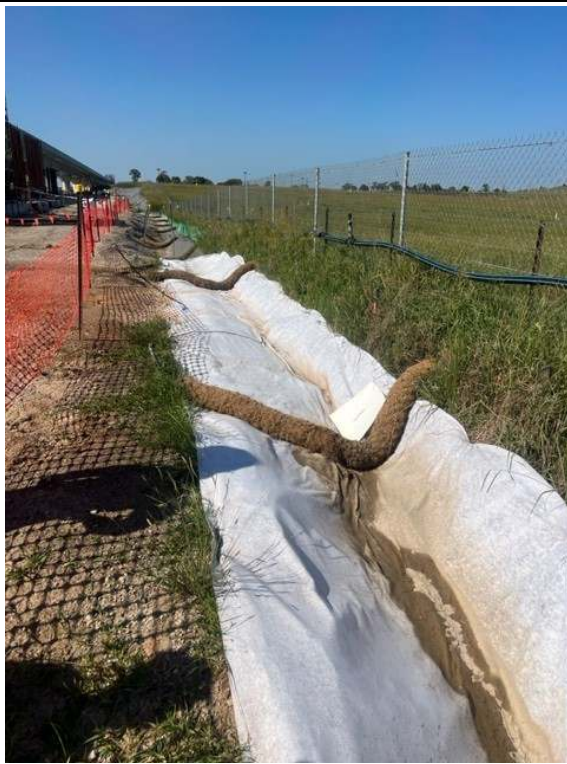
Photos 13 & 14: Swales had been established and controls were in place to filter the flow of stormwater from the site to the sediment basin
