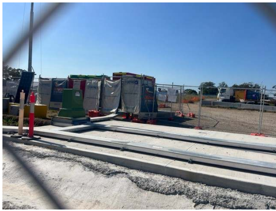
Photo 11: Noise blankets in place around generators
