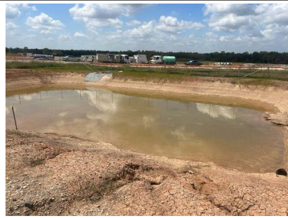
Photo 32: Sediment basin in place and in use for dust suppression
