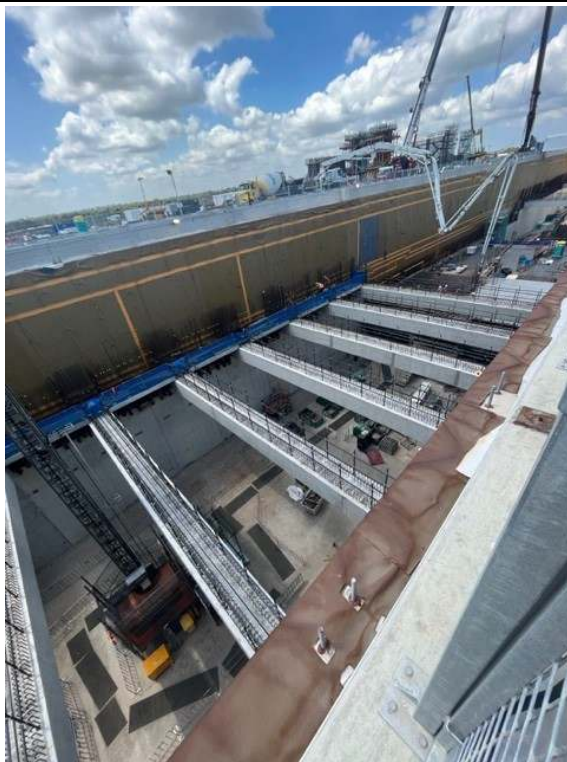
Photos 29 & 30: Beams had been installed on the top of the station box and a concrete pour was underway
