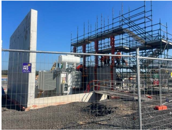
Photo 7: Substation construction underway, including transformer filling
