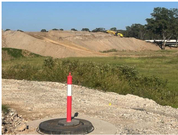
Photos 3 & 4: Stockpile of site-won VENM being relocated to an area adjacent to the future permanent basin.
