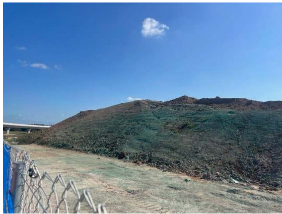
Photos 15 & 16: A large stockpile was in place and was stabilised with polymer and controlled with staked straw bales, vegetation growth and a sediment fence
