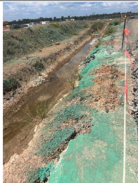
Photos 33 & 34: An open swale has been established to divert water around the site and was fitted with rock checks to filter and slow flows. PLM advised floc blocks were installed at check points during high flows to further reduce sediment load
