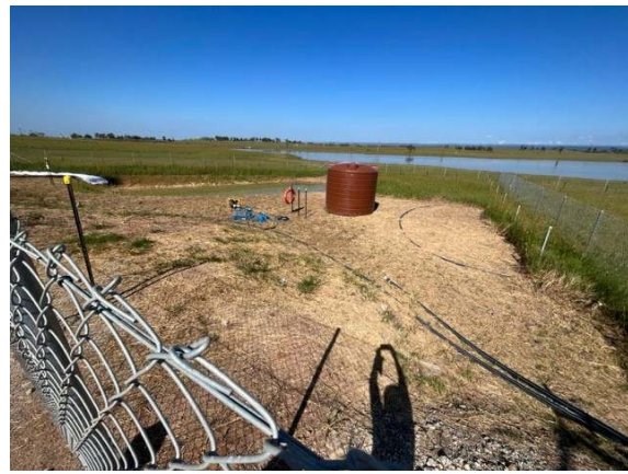
Photo 12: Water from the sediment basin was in use for dust suppression
