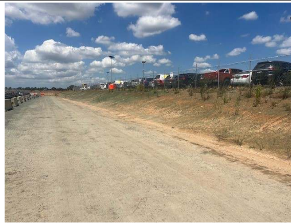
Photo 31: The internal access road was well-stabilised and batters were sprayed with polymer. Minor rill erosion was present but was being monitored.
