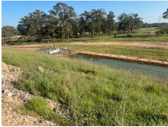
Photo 1 & 2: Temporary sediment basin in place. Water from this basin is pumped to the main sediment basin as required prior to testing and reuse on site for dust suppression.
