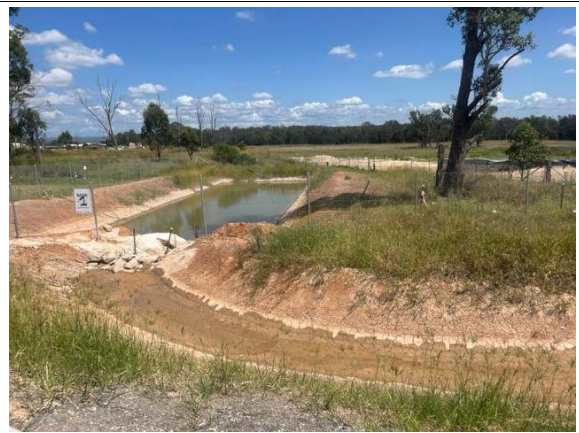
Photo 26: A stabilised swale was in good condition and flowed into a sediment basin, which had not yet been utilised
