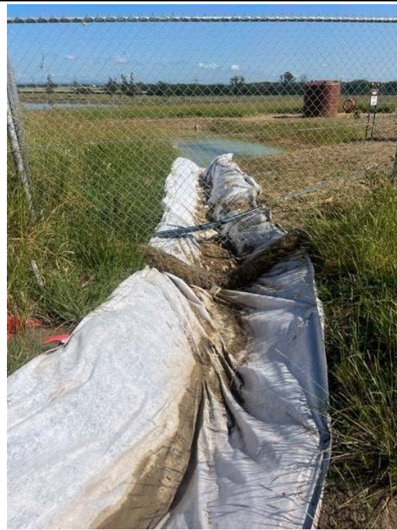
Photos 13 & 14: Swales had been established and controls were in place to filter the flow of stormwater from the site to the sediment basin
