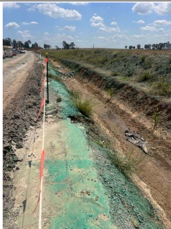
Photos 33 & 34: An open swale has been established to divert water around the site and was fitted with rock checks to filter and slow flows. PLM advised floc blocks were installed at check points during high flows to further reduce sediment load
