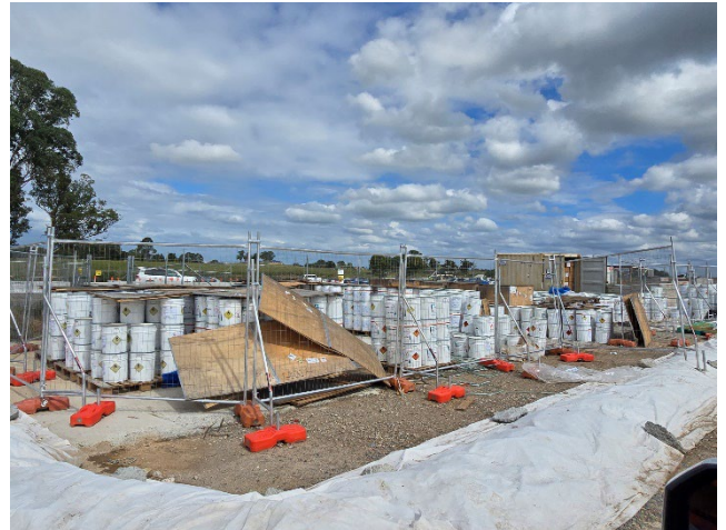
Luddenham to M12 – Bunding of flammable materials in storage laydown area.
