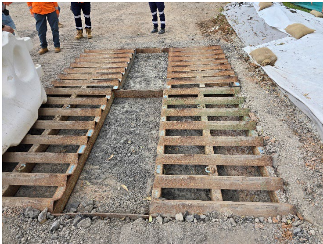
BSF - Rumble grids were installed.
