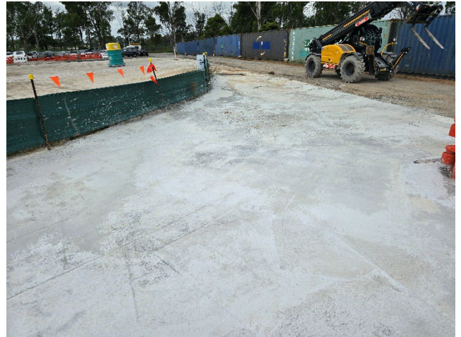
BSF – Concrete washout bay was sealed.
