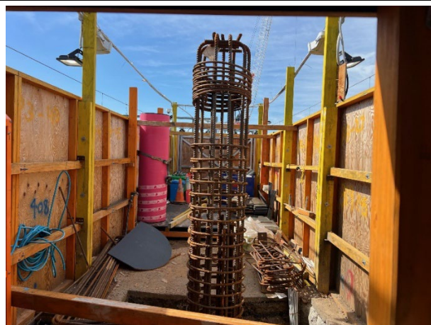
Platform 3/4: Pile cages are in place on platform 3/4 awaiting concrete pours.
