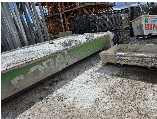
BRD – Concrete washout on stabilised area.
