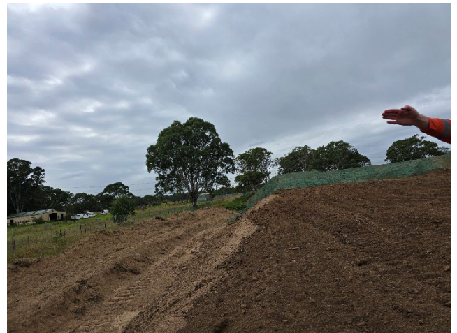
SMF – Polymer spraying of the topsoil stockpile had commenced, weed maintenance at the rear of the stockpile required attention.
