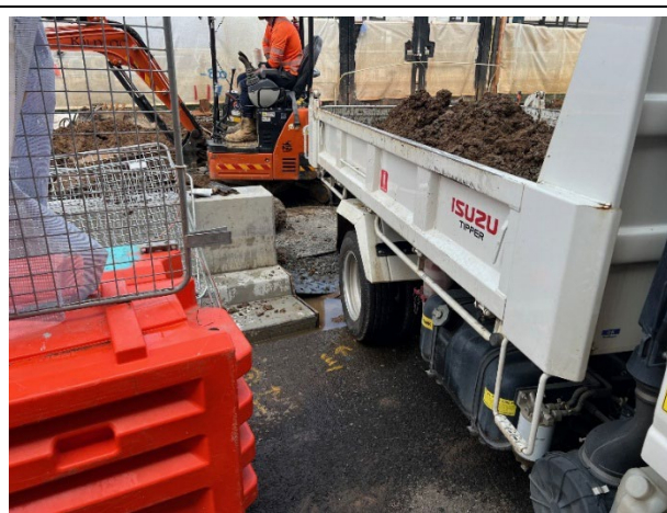
Road between site and carpark: Trucks loading out from the compound area were not driving on mud, keeping their wheels clean.
