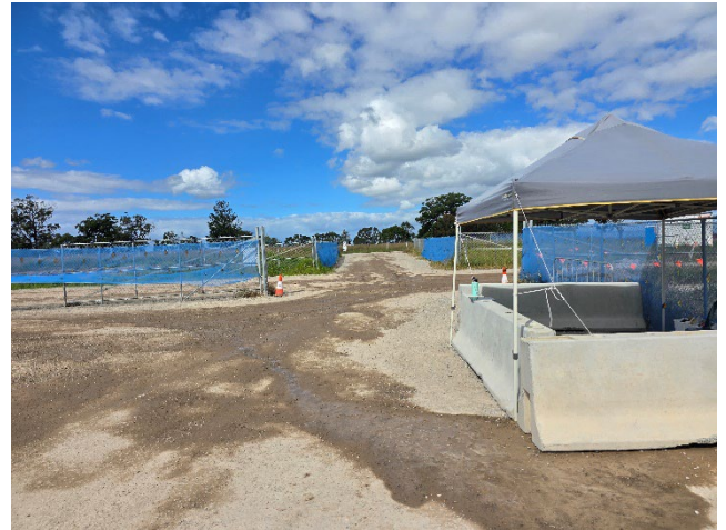
LUD – Light vehicle (LV) and haul road interface stabilisation was pending. Increased use of water carts and street sweeper was ongoing to control sediment tracking.
