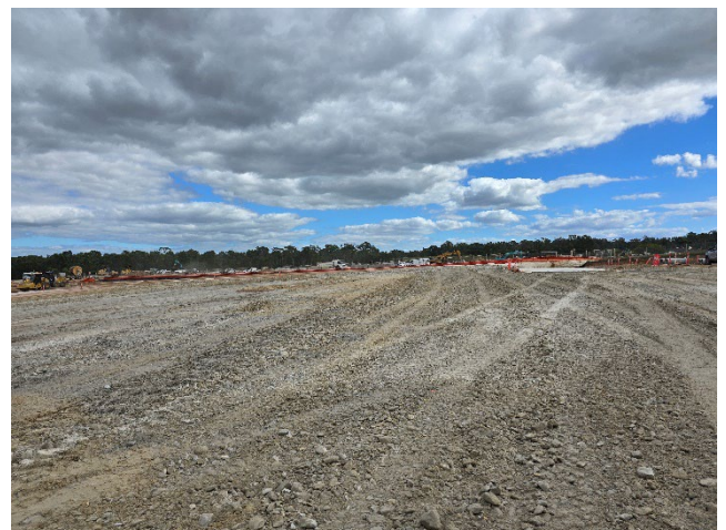
BRD – Compaction for the permanent car park.
