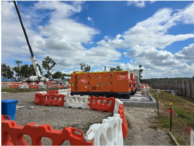
BSF – Larger generators were being commissioned (noted to be quieter as under less load than smaller generators).
