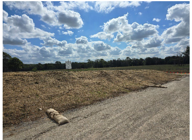
BSF - Hydro-mulch on topsoil batter and ESC checks on toe of batter.
