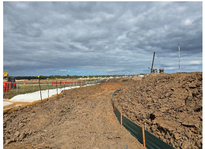
BRD – Topsoil stockpile removal continued, ESC was maintained. Rear of stockpile graded to pool onsite.
