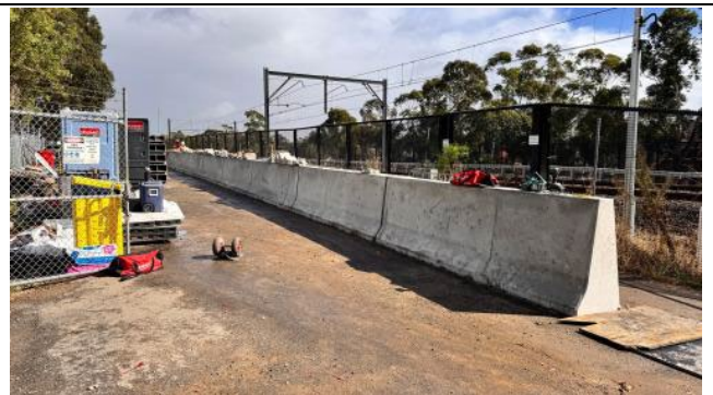
Figure 6 – Punchbowl - Concrete barrier works underway
