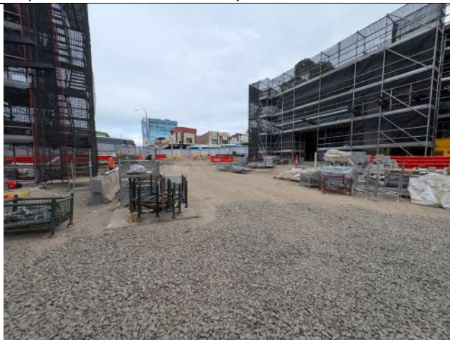
Figure 9 – Bankstown - Majority of CSR works complete, site has been stabilised with ballast to minimise dust generation
