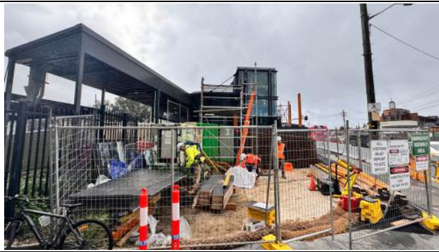
Figure 7 - Canterbury Road – Footpath works near Canterbury Signal Hut ongoing, works on overbridge to recommence shortly mainly in the form of remediation works leading up to concrete barrier works
