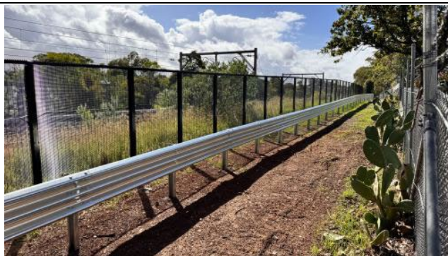
Figure 5 – Punchbowl - Steel barrier installation complete near The Boulevard. Concrete barrier works underway
