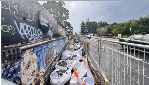
Figure 1 – Illawarra Road – Ongoing footpath excavation and utilities relocation ahead of concrete barrier works, partial footing demolition, once Photo Archival Recording has been completed
