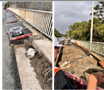
Figure 4 – Stacey St overbridge - FRP and excavation works underway
