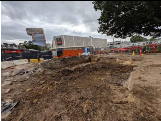
Figure 7 – Bankstown - Onsite Detention (OSD) tanks installation excavation ongoing. It is understood that asbestos containing material (ACM) was identified during this excavation which was removed for offsite disposal to a licenced facility
