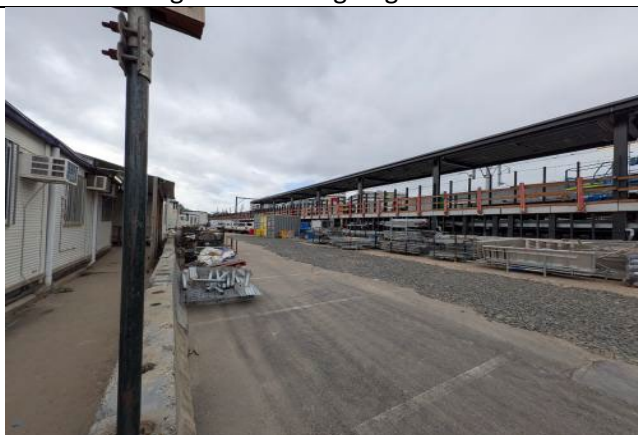
Figure 5 – Bankstown Station - Laydown area in operation. Ballast cover in place to minimise dust generation. Hardstand area was observed to be dirt free.
