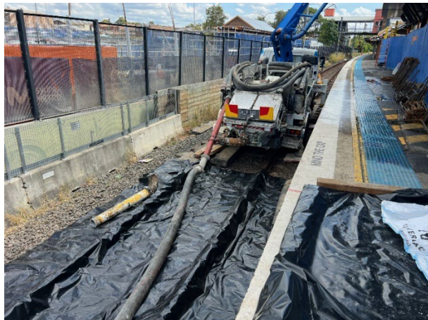
Platform 3/4: HDPE plastic was laid out to capture any leaks along the concrete pump line.
