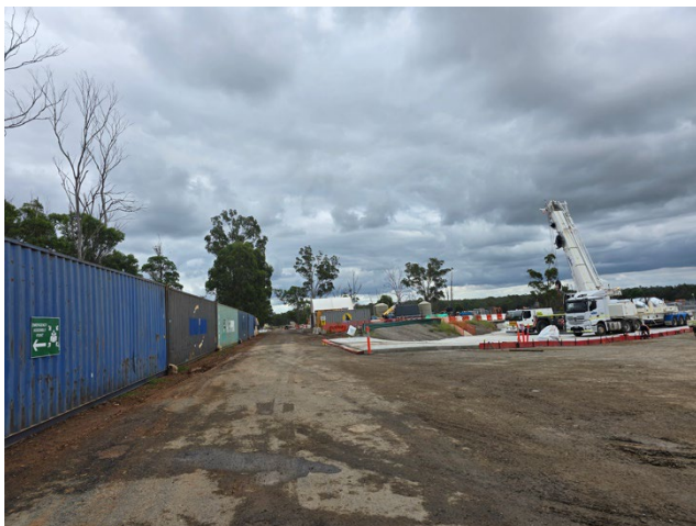
BSF – Concrete crane pad installed; PLM indicated that stabilisation of the haul route was to be completed over the coming weeks.
