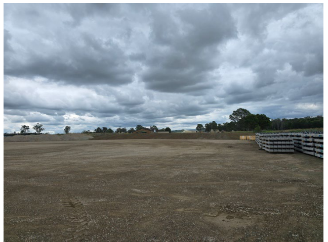
BSF – Topsoil stockpiles had some seed placed (minimal growth), and PLM indicated that hydroseeding was scheduled at the end of the month. Additional ESC checks along base of the batters were suggested to minimise erosion.
