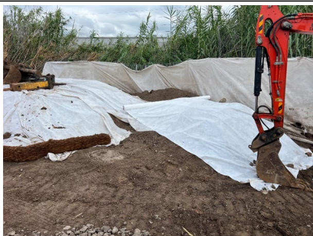
MAF1: ERSED controls required proper installation and pinning to suit the volume of material.
