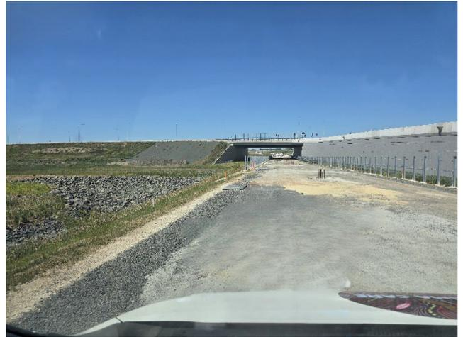
**Portion 4** – GST construction continued through Portion 4 towards Portion 5 on the right. Rock check swale and retention basin to the left.
