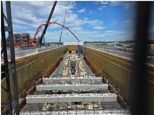
**BRD** – Station box showing beam installation and concrete pour.
