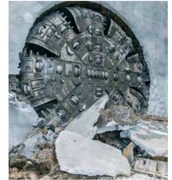
TBM2 Florence was the last mega borer to finish work
