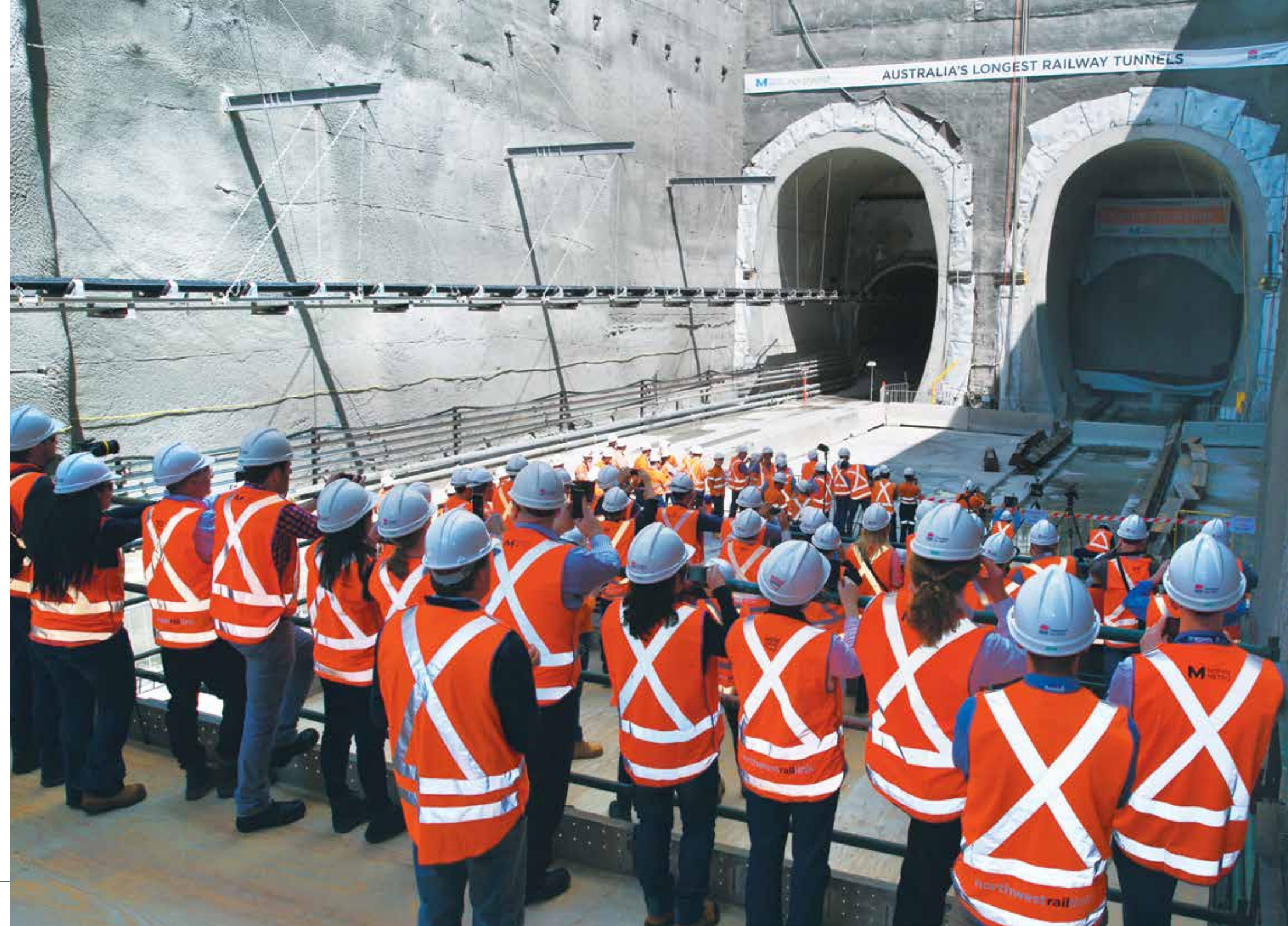
Community members watch TBM2 break-through at Castle Hill, 2 October 2015
