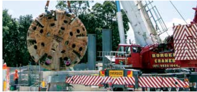
TBM4 Maria cutter-head retrieval at Epping, 23 November 2015
