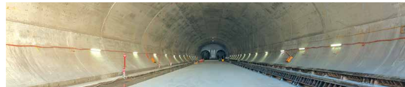
Crossover cavern interior, September 2015
