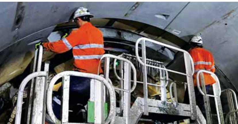
Workers installing segments underground on TBM1 Elizabeth, December 2014
