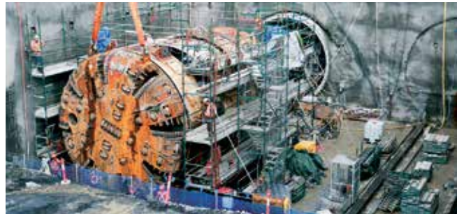
TBM1 Elizabeth cutter-head retrieval at Cherrybrook, 7 January 2016
