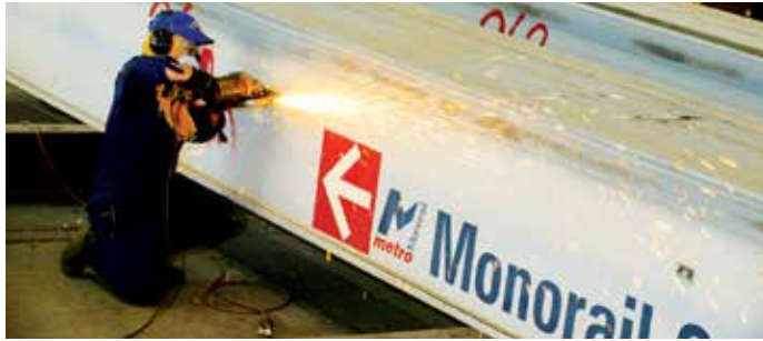
Recycling Sydney's monorail beams, February 2014
