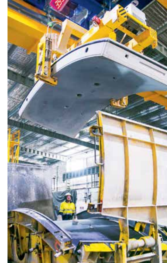
The last concrete segment, November 2015
