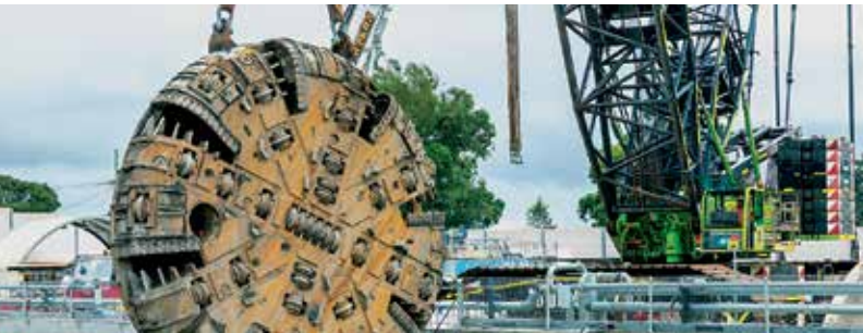
TBM2 Florence cutter-head retrieval at Cherrybrook, 6 February 2016
