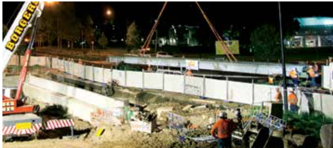
Monorail being installed at Norwest, April 2014
