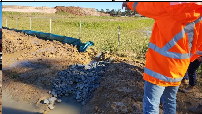
SMF – tie-in works with SMF were ongoing. Stabilisation of the channels was pending access due to wet conditions.
