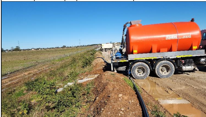
SMF – water tankers moving site water to the sumps were noted to be causing embankment erosion. Operators were tool boxed and batters stabilised.
