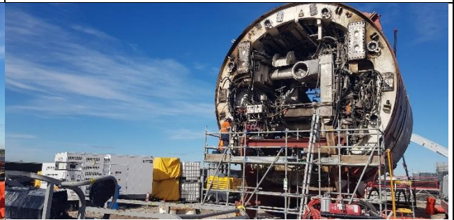
Aerotropolis view south east – TBM shield preparation for transport.
