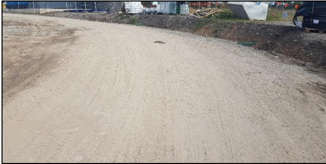
Bringelly – Soil accumulations on sealed internal haul roads.
