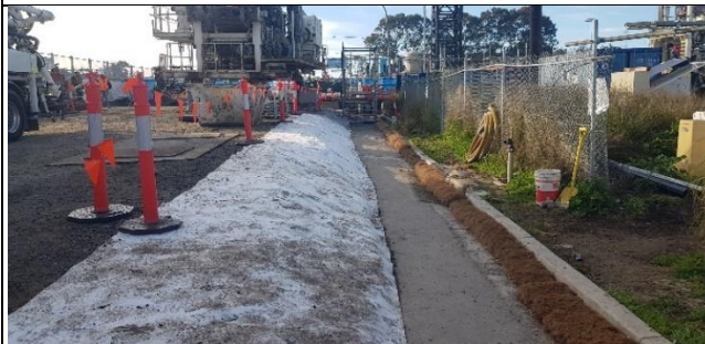
St Marys south side of Station St view east – erosion and sediment control measures significantly improved.
