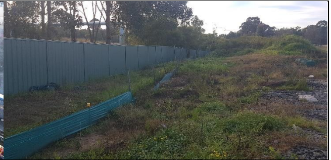
Orchard Hills Northern boundary – Sediment fence required repairs.
