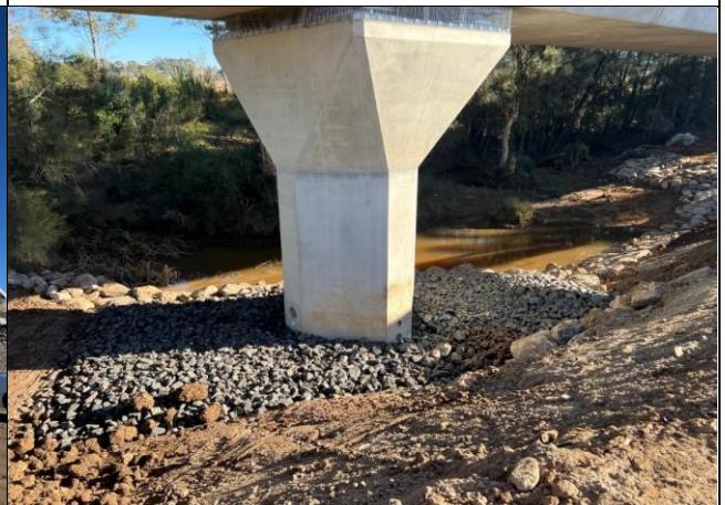
Blaxland's Creek - Scour rock has been placed around the base of the piers
