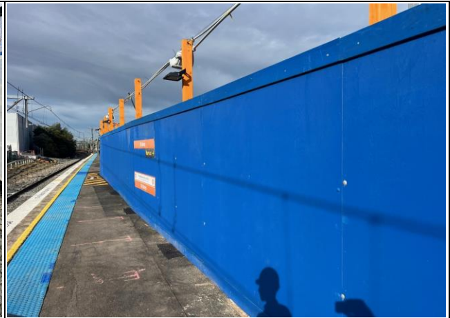
Platform 1/2 - Hoarding has erected on the platform sealed at the base to prevent water from running onto the public standing area
