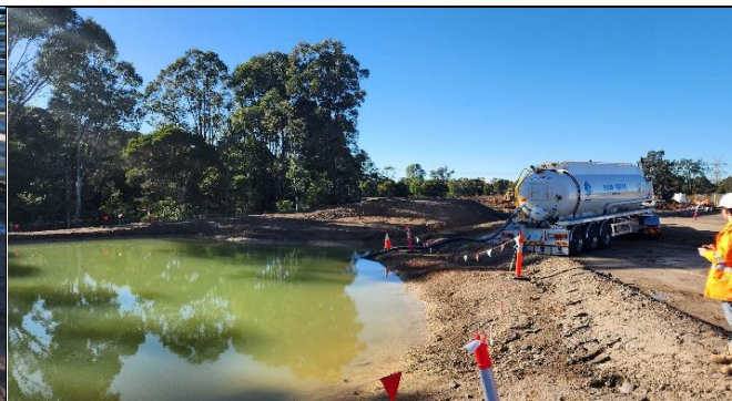
ORH –Turkey nest being emptied via tankers to STM water treatment plant.
