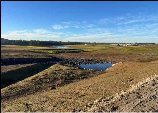
Elizabeth Drive Compound - Batters have been completed and are now hydromulched
