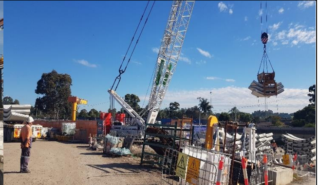
Claremont Meadows shaft view north – Final delivery and tunnel segment craning into shaft.
