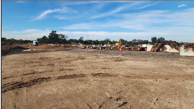
ORH –concrete batch plant - preparation for concrete base slabs had commenced, it was noted that large areas were exposed in preparation for slab pours.
