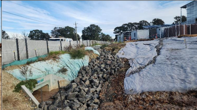
ORH – Maintenance of ESC and removal of sediment from internal swale was ongoing – rock added to eroded sections, but tie in work was ongoing
