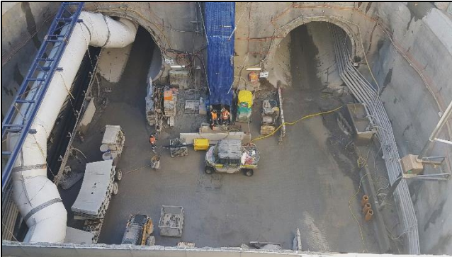
Claremont Meadows shaft, view north – Shaft activities with one air extraction/spoil conveyor system left.
