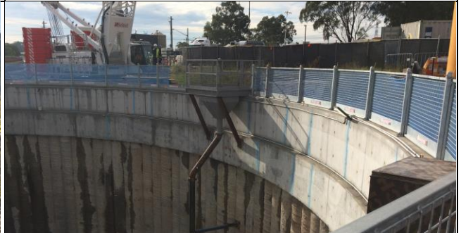
Claremont Meadows shaft view northeast – Concrete delivery drop-pipe.
