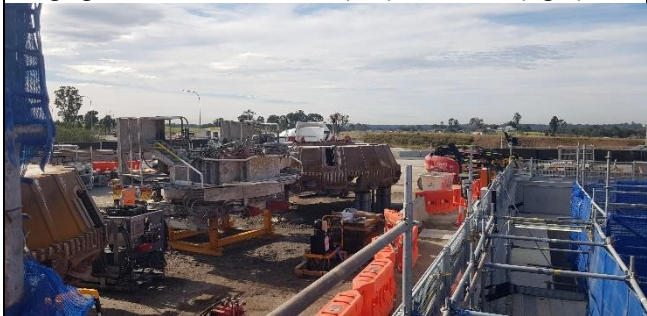
Aerotropolis view west – TBM cutter head preparation for transport.
