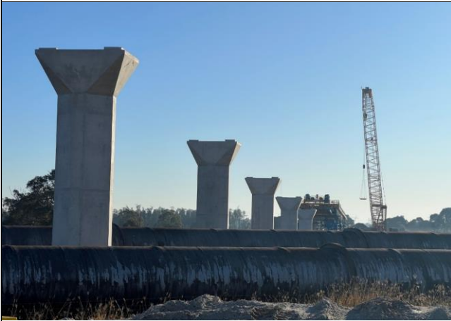
Luddenham North - Piers and the gantry are ready for viaduct installation over the Warragamba pipeline in July
