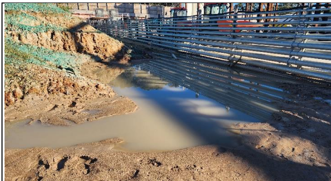
ORH – Maintenance of the Erosion and Sed. Controls (ESC) to the sump was not actioned
