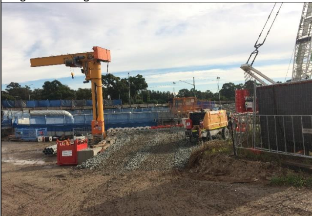
Claremont Meadows view northwest – Concrete deliveries ramp to drop-pipe.
