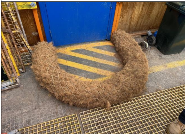
Platform 1/2 & 3/4 - A coir log has been used to control runoff adjacent to the main access door
