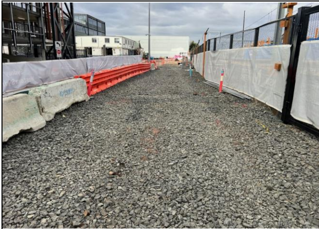
Compound - The ballast accessway is clean and extends from edge to edge, reducing the mud tracking risk
