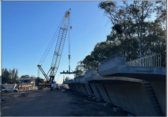
Defence - Viaduct elements are stored within the site awaiting lifting into place
