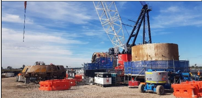
Aerotropolis view east – TBM retrieval and dismantling staging area with cutter head (left) and shield (right).
