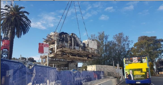
St Marys view south east – TBM Bridge lift to TBI area.
