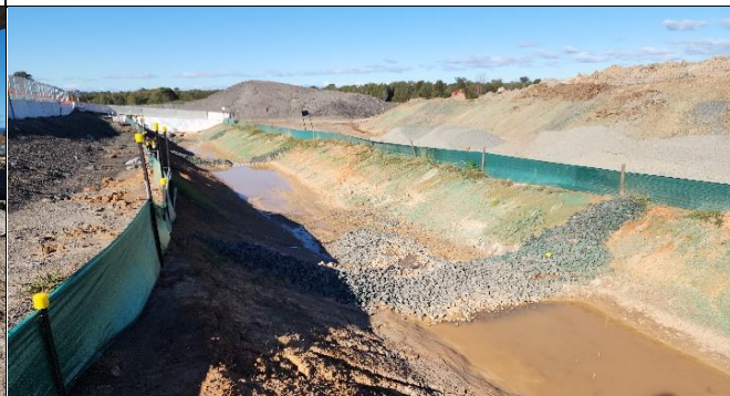
AEC – Up-stream water diversion with rock checks and inline flocculation.
