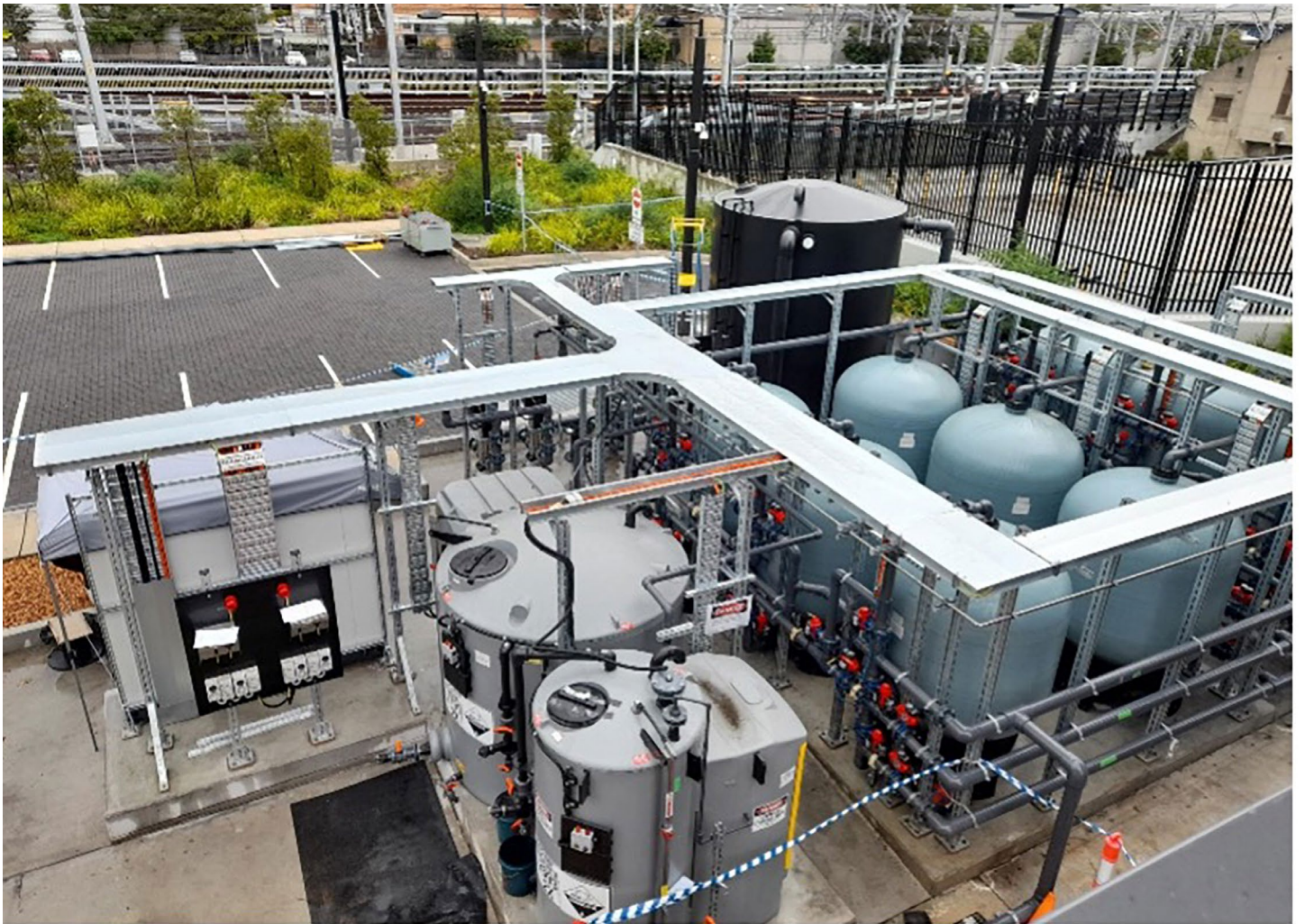
The new water treatment plant combines sustainable outcomes with excellence in construction
