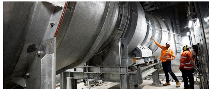
Two of a total of 72 large tunnel ventilation fans needed to operate the extended network are housed in the Northern Dive Services Building.
