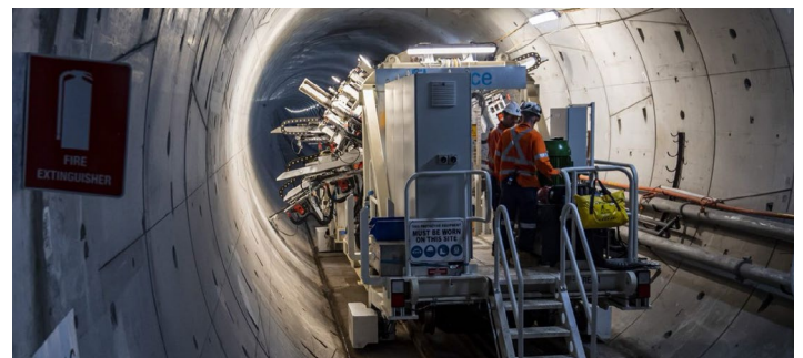
Custom made equipment was used to safely and efficiently drill more than 300,000 holes in the tunnels as part of the City & Southwest tunnel fitout.
