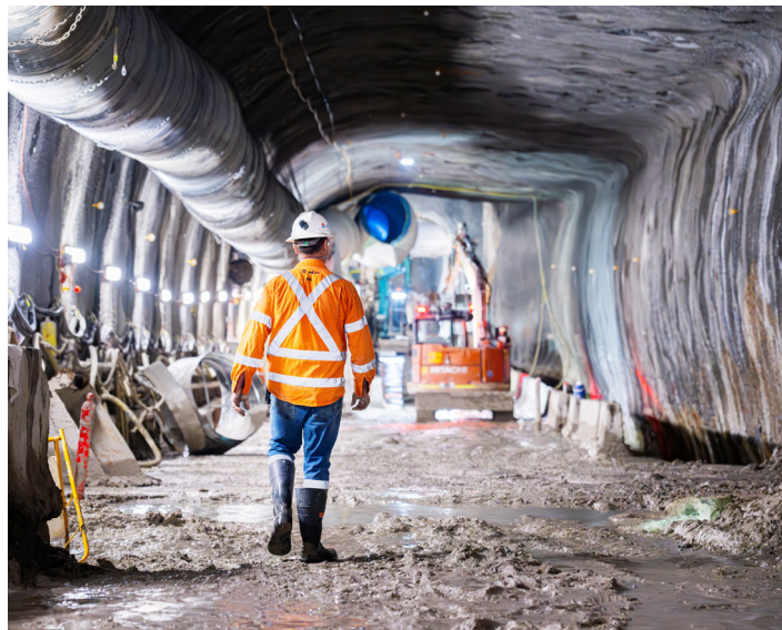
Two roadheaders are being used to excavate the turnback tunnels.
