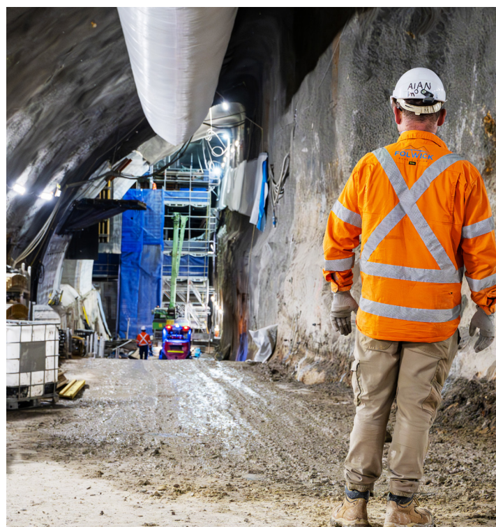
The station cavern is being excavated in three stages.
