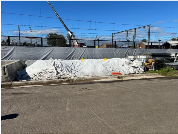
Compound – Retained material at the compound has been wrapped in geofabric
