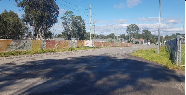
Claremont Meadows – Negligible tracking noted from southern site access onto Gipps Road.
