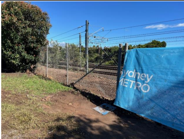
Hobart St – The westerly stockpile along Hobart St has been removed
