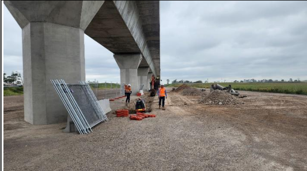
LUD – Removal of drainage for upcoming piling work
