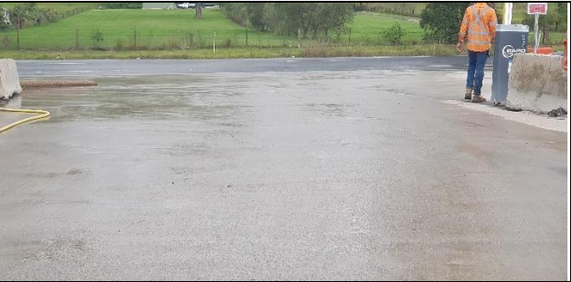
Orchard Hills exit – Exit apron free of tracking.
