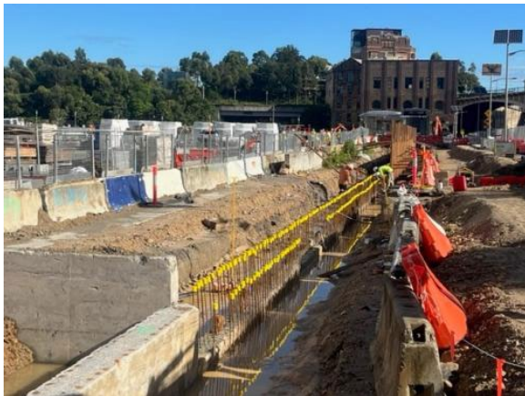
Retaining wall construction in Zone 3 was ongoing.
