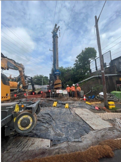
Piling for a crash beam re-commenced at Victoria Road bridge, Marrickville. ERSED controls were well established in the flood zone.
