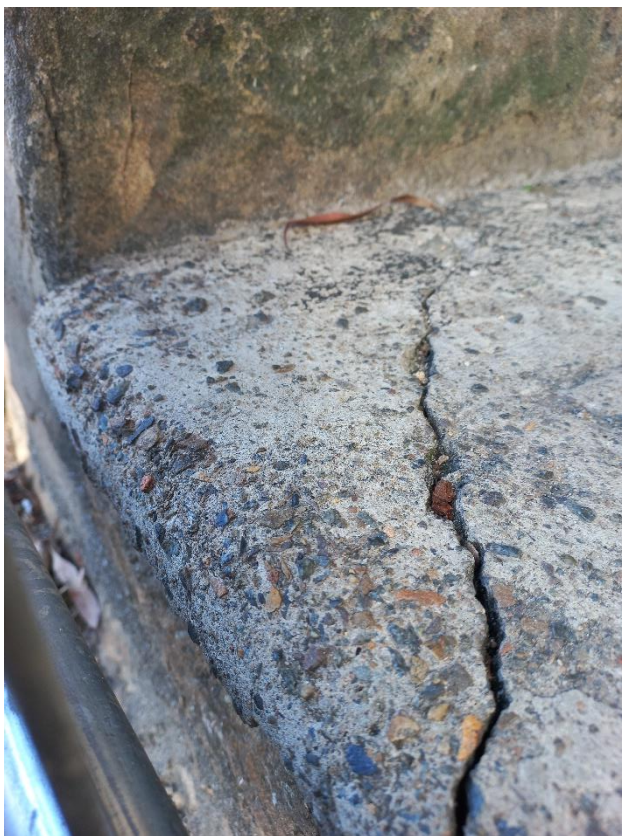
Figure 2: Small pebble aggregate and cracking at the edge of the landing.
