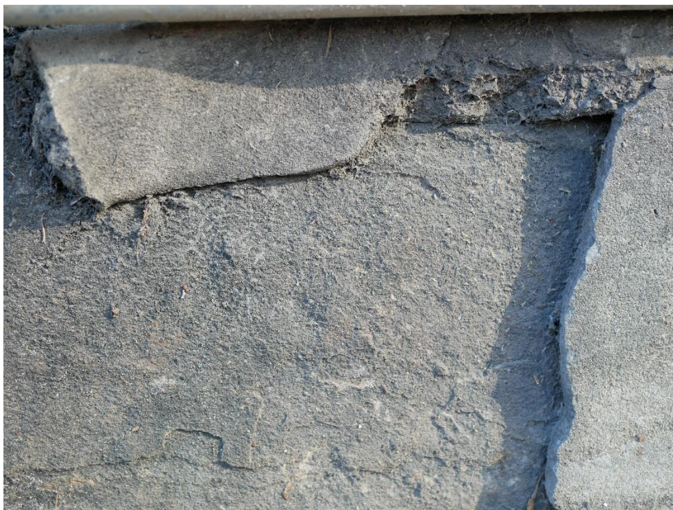
Figure 4: The remaining render on the Hickson Road face of the landing step does not appear to be original and has no aggregate.
