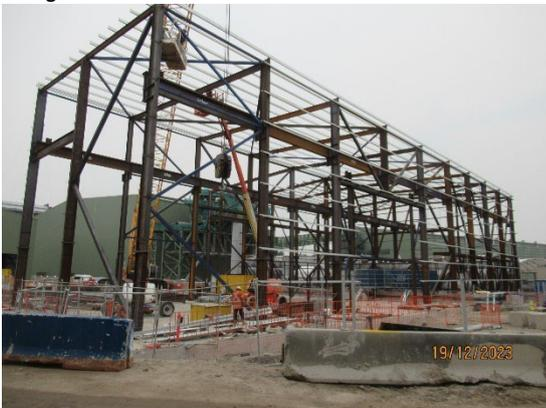
Figure 3.7 The Bays: Frame being constructed for the Segment Shed over the station box
