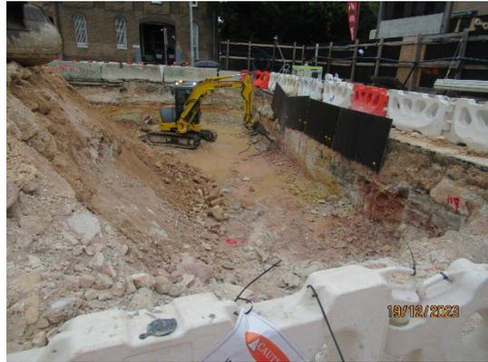
Figure 3.4 Pyrmont West: Hammering of sandstone adjacent Paternoster Row as part of retaining wall works.
