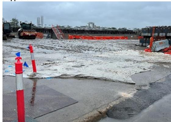
Figure 2.14: Clyde MSF Site – inadequate erosion and sediment controls during the rainfall event on the 2012/2023
