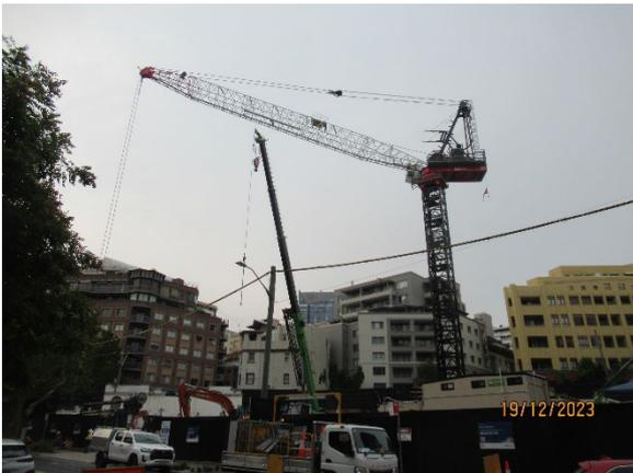
Figure 3.1 Pyrmont East: Diesel powered Tower Crane installed and operating.
