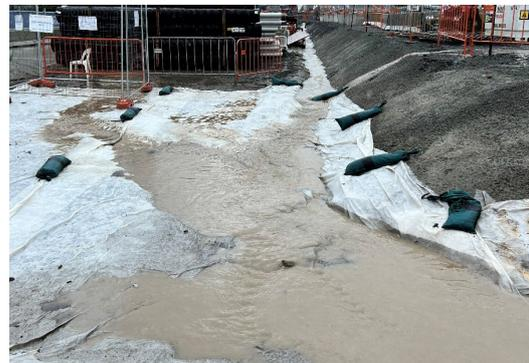
Figure 2.6: Clyde Dive site – sediment controls during rainfall on the 20/12/2023
