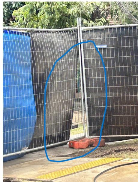
Figure 4.2 Westmead Utility Works: Noise blanket gaps during day works.
