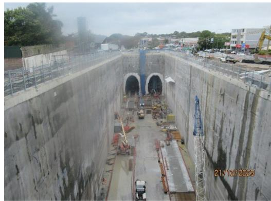
Figure 1 4 Station Box excavation completed (Burwood North). FRP for TBM plinths.
