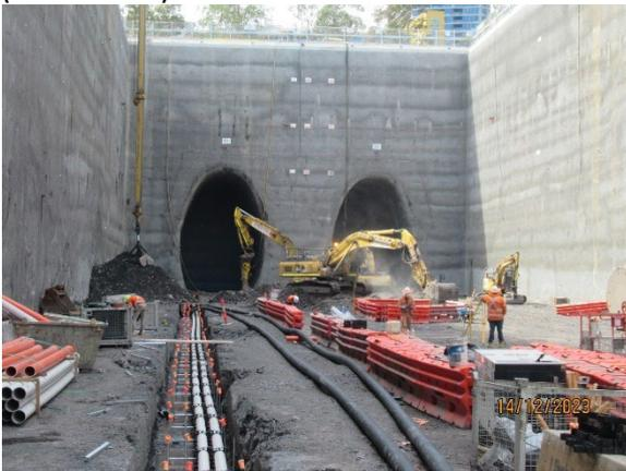
Figure 1.7 Excavation completed. Last of spoil being removed. Services installation (SOP)
