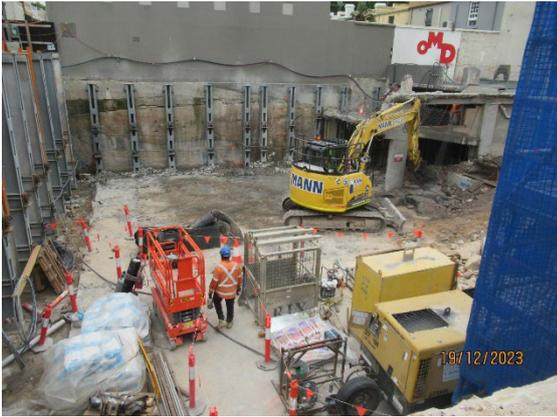
Figure 3.3 Pyrmont West: Ongoing works to install wall support around former basement. Removal of concrete slabs.
