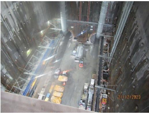
Figure 1 1 Tunnels at western end of the station box (The Bays).
