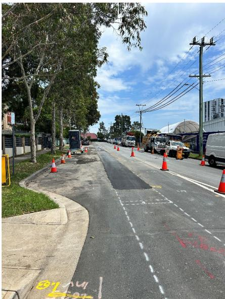
Figure 4.1: Westmead Utility Works - Bailey Street following conduit installation
