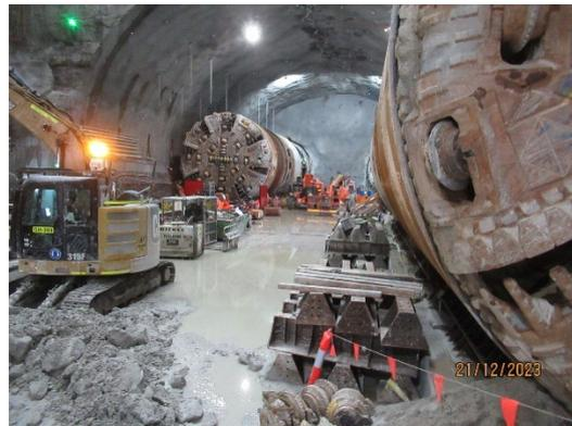
Figure 1 2 TBMs in the Eastern Shaft (Five Dock).
