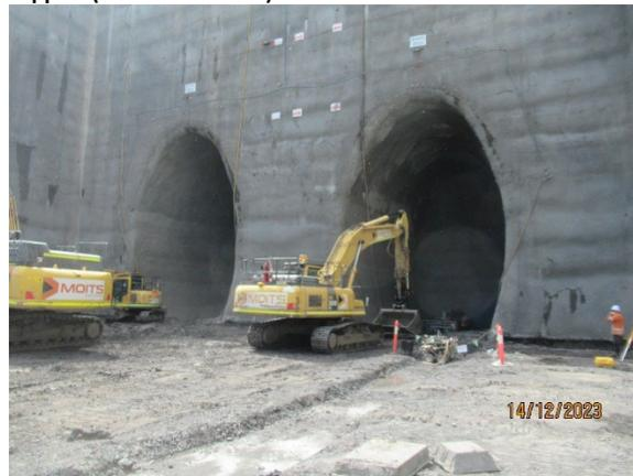
Figure 1.8 Services trenches being excavated in front of the nozzles (SOP).
