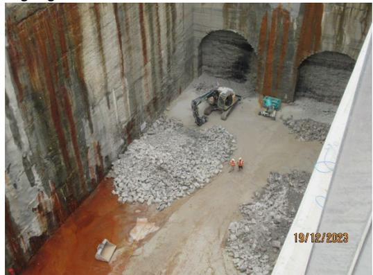
Figure 3.8 The Bays: Niches excavated from the wall of the station boxes for TBM operation
