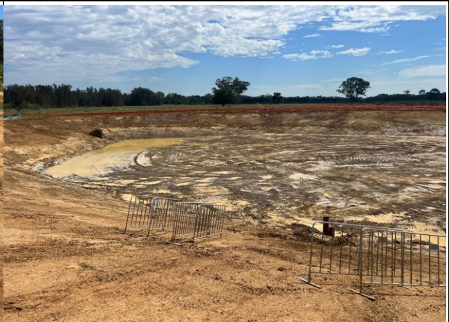
Cosgroves Creek – Work continues on excavating the 30ML flood retention basin
