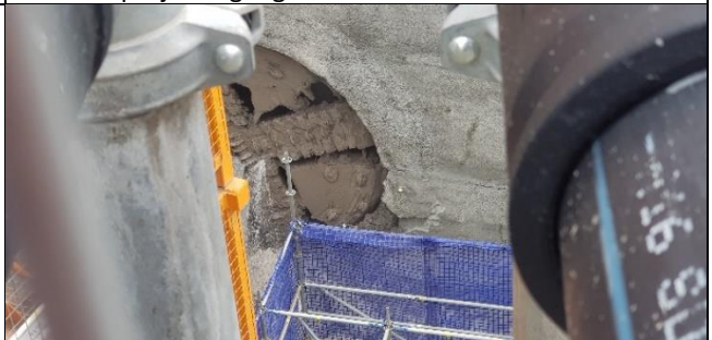
Claremont Meadows: TBM Catherine breakthrough.
