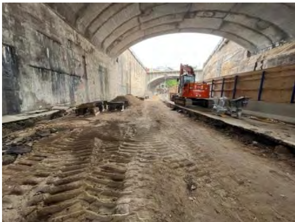
Demolition of kerb, gutter and road under heritage bridges, Hickson Road North.
