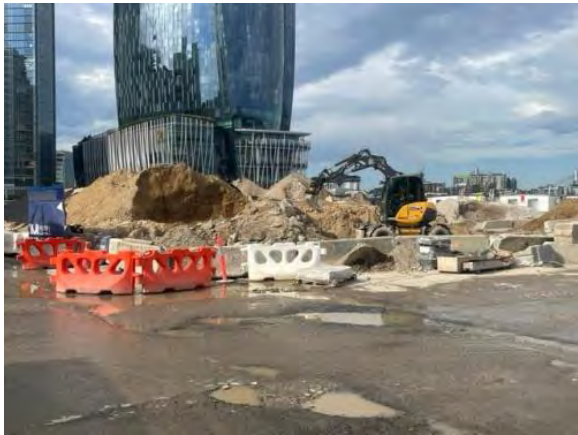
Remaining stockpiles in use for backfill, and hardstand wet, reducing dust potential.
