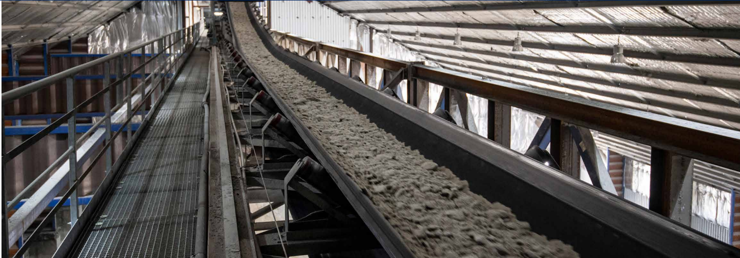
Image: Conveyor belt. Spoil storage and removal Marrickville Dive site.
