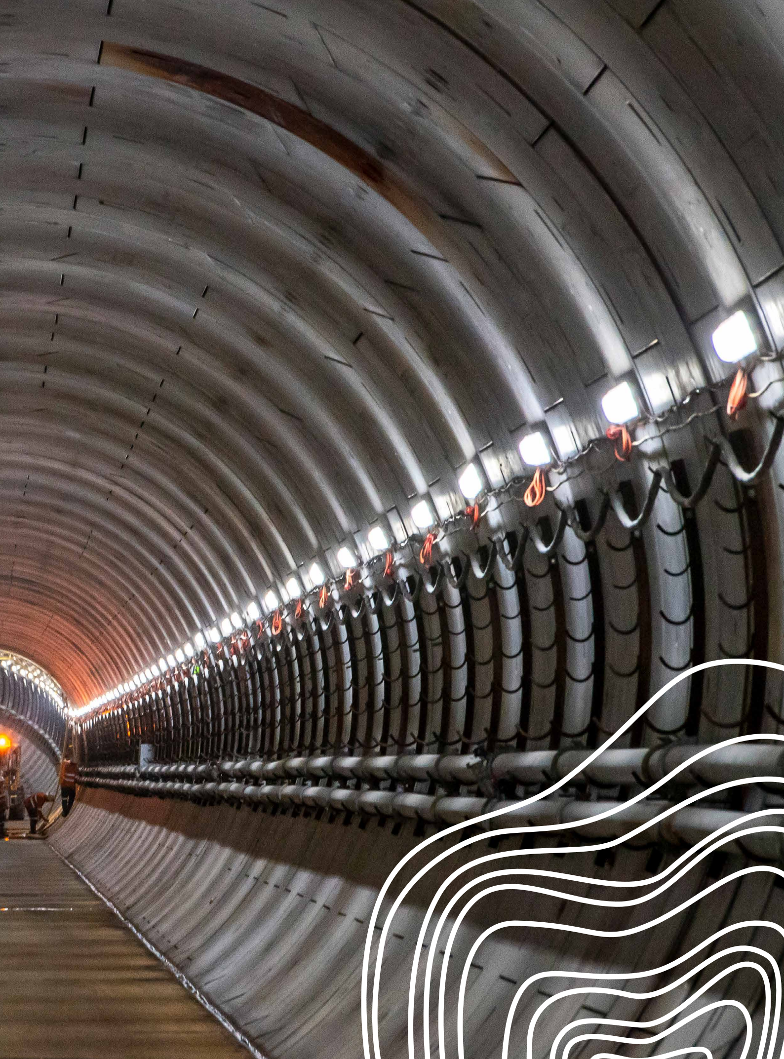
Image: Tunnel under Sydney Harbour.
