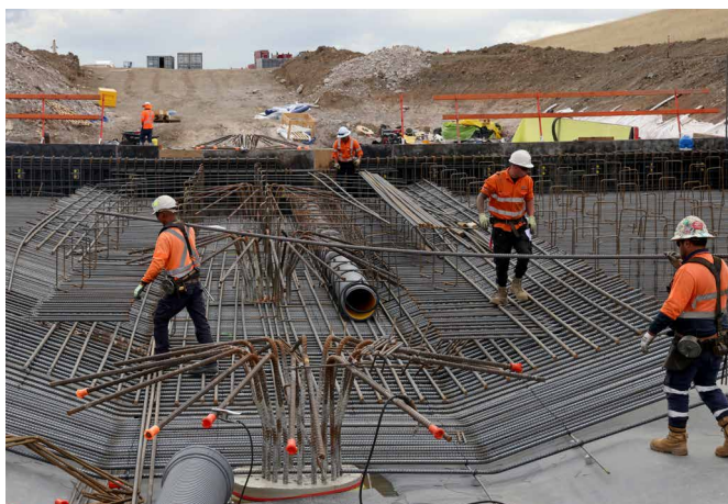
Image: Establishment of site at the Sydney Metro Western Sydney Airport project.
