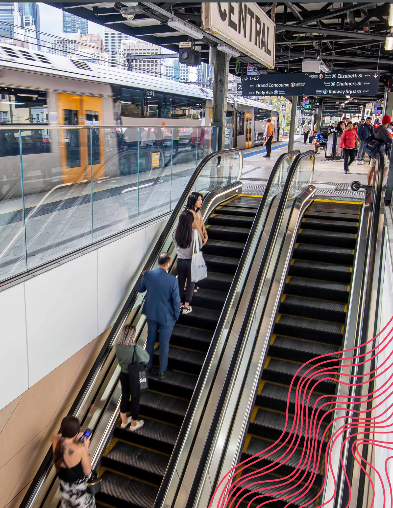
Image: In preparation for Metro services at Central Station escalators have been installed to provide convenient access to suburban platforms.
