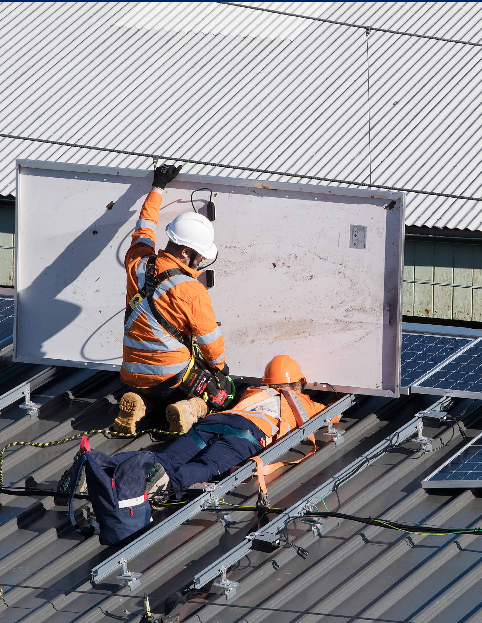
Image: Solar panels are being installed as part of Sydney Metro's major upgrade of Central Station.
