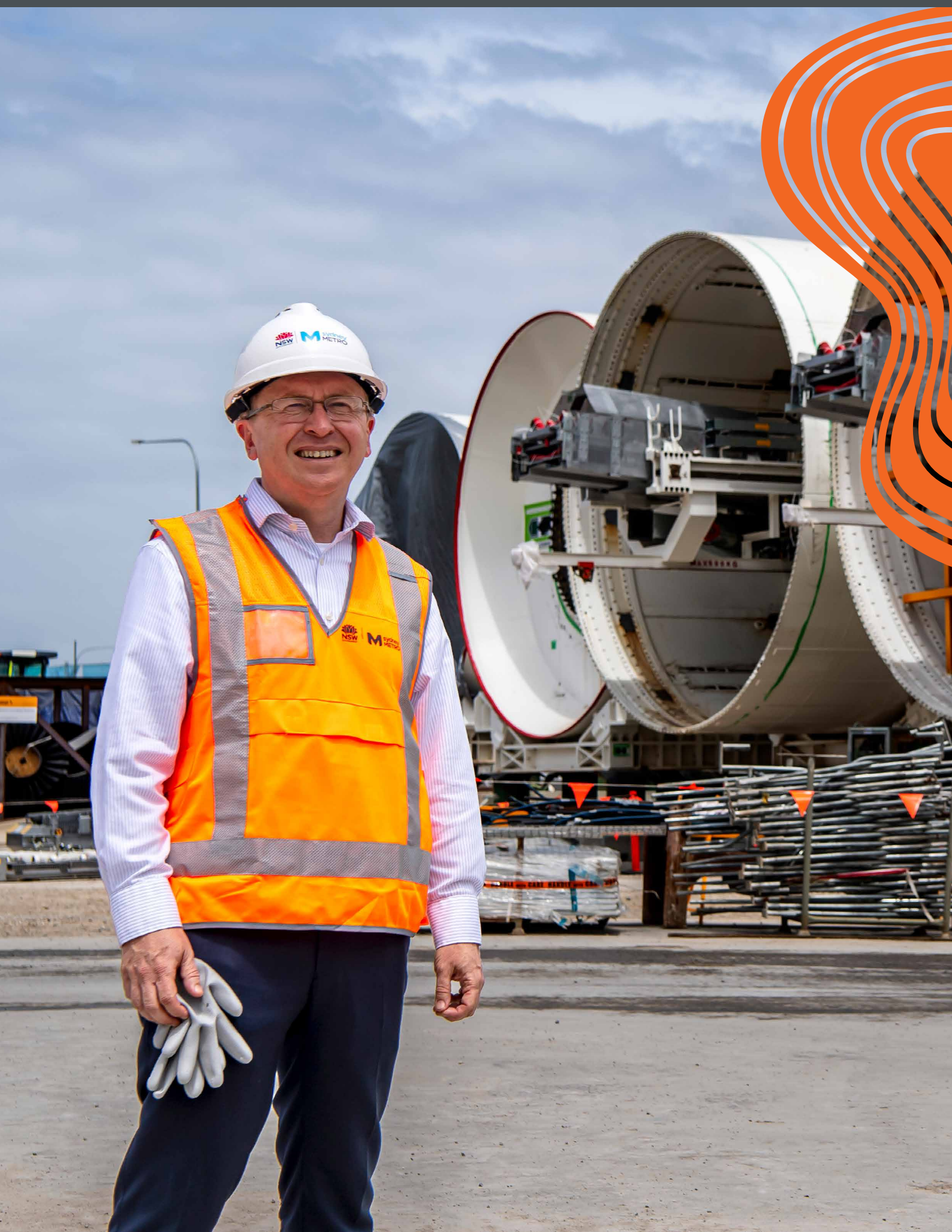
Image: Sydney Metro Chief Executive Peter Regan visits The Bays station site to view the progress on the station box/dive site and the tunnel boring machines waiting to be launched.
