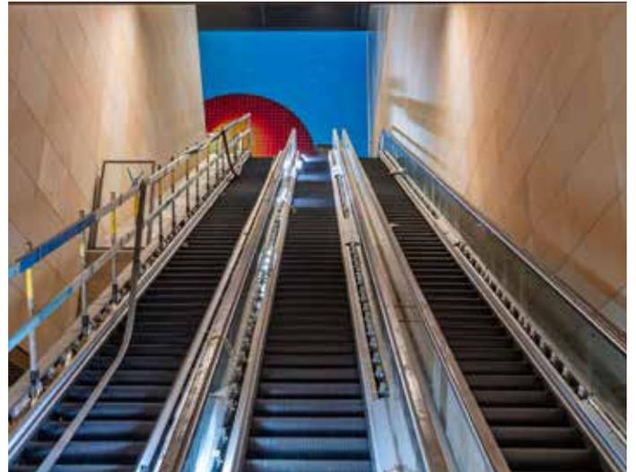
Gadigal Station's ten escalators have all been installed. Technicians are now working to prepare them for operation, which includes connecting power, installing treads and programming their speed.
