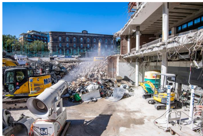
An example of a water cannon being used during demolition work at our Pyrmont site
