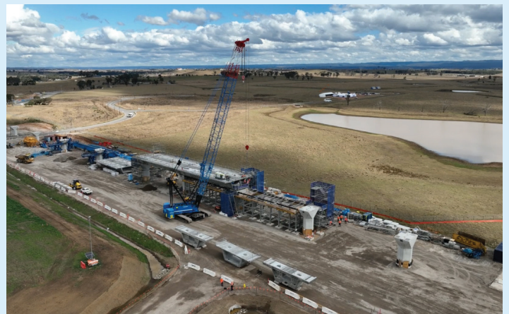
Installing viaduct segments for the new Luddenham Station.
