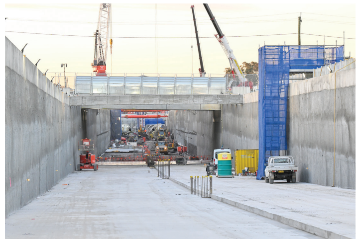
The Orchard Hills dive structure looking south towards the Lansdowne Road bridge, will allow excavation to continue underneath Lansdowne Road.
