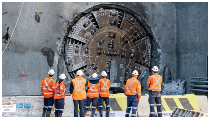
TBM Peggy breakthrough at the Airport Terminal site in late August 2023.
