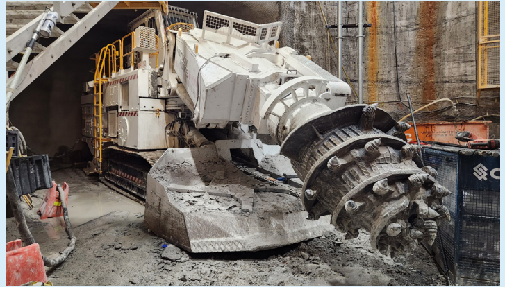
Roadheader at Clyde
