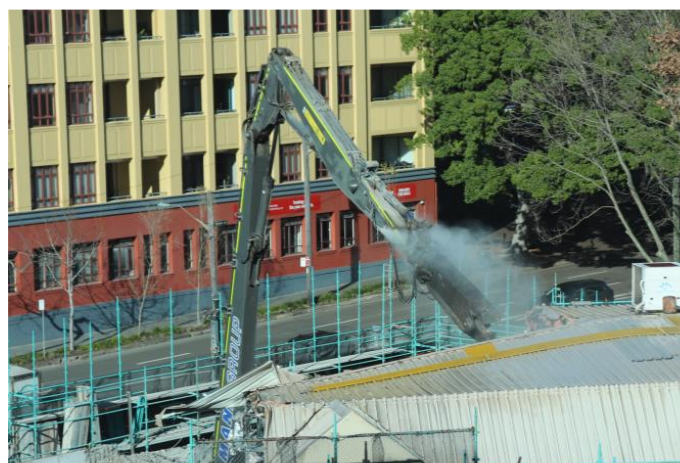
An example of a pulveriser and water mister attachment being used during demolition work at our Pyrmont site
