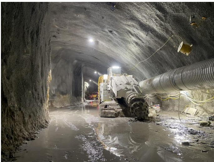
An S300 roadheader inside the Hunter Street station cavern
