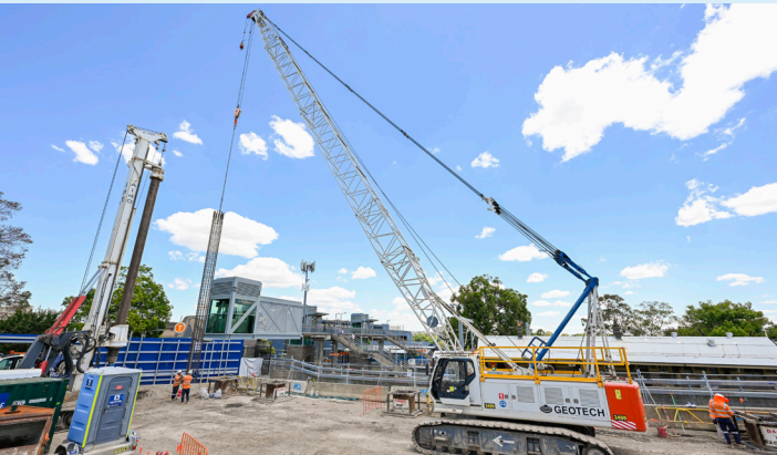
A piling rig at the North Strathfield metro station site.
