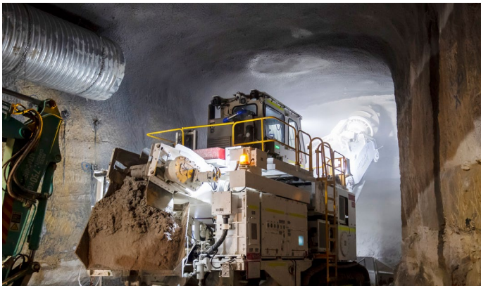
An image of the S300 roadheader inside the Hunter Street decline access tunnel
