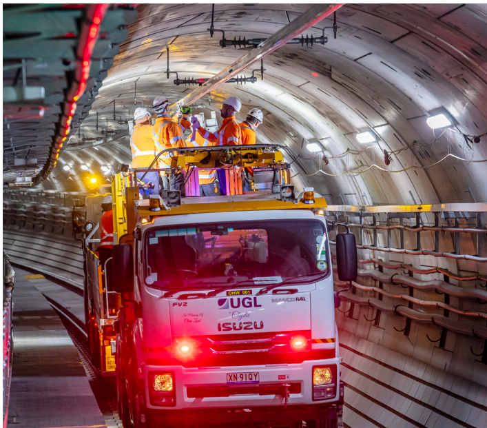
Workers under Sydney Harbour installing the overhead wiring needed to power the driverless Metro trains
