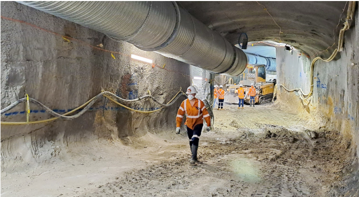
Roadheaders at work excavating the temporary decline tunnel at the Hunter Street Station site
