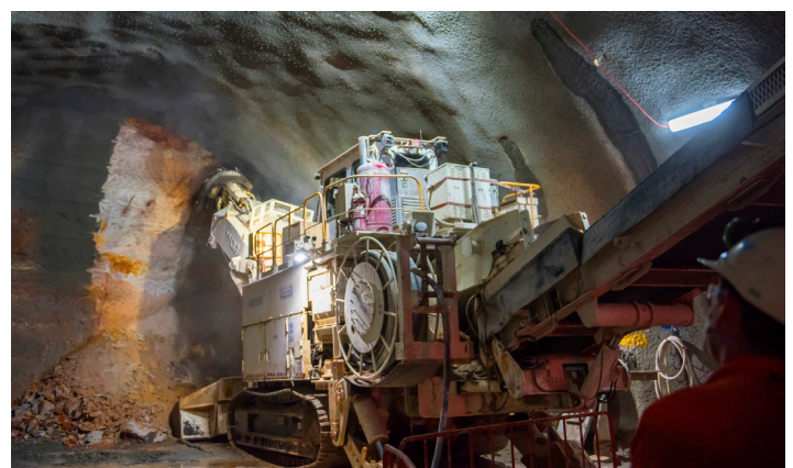
Roadheaders are used to excavate underground structures that are different shapes and sizes
