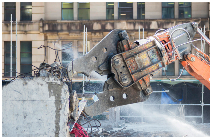
Pulverisers and shears (pictured) are used to make demolition much quieter
