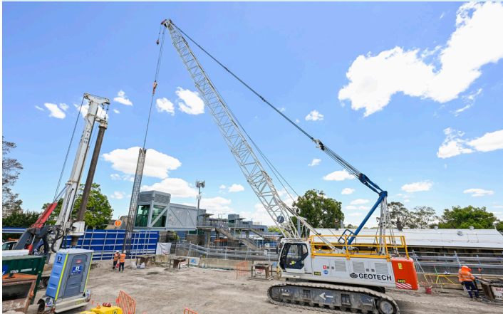
A piling rig at the North Strathfield metro station site.
