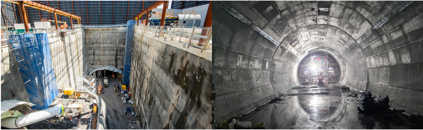
Entrances to the underground pedestrian tunnel (left) and crossover cavern (centre) are located inside the excavated station box. Underground pedestrian tunnel.
