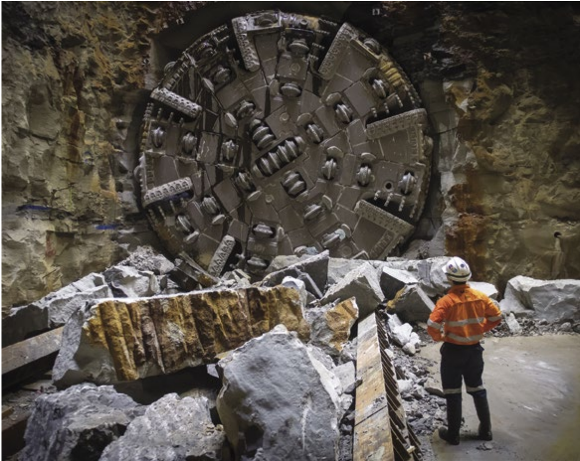
TBM 3 Wendy, dug a 6.2-kilometre tunnel to the edge of Sydney Harbour, on the City & Southwest project.
