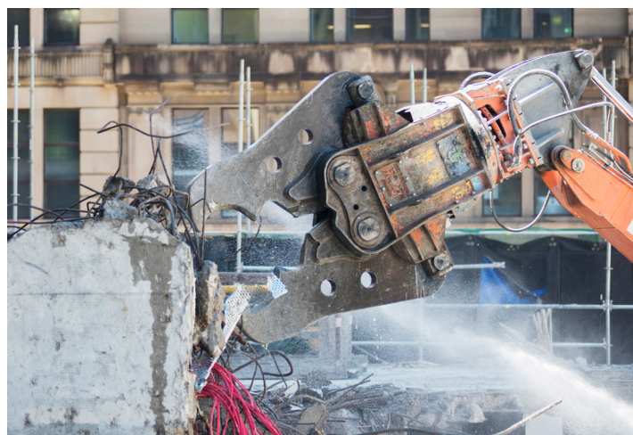
Pulverisers and shears (pictured) are used to make demolition much quieter
