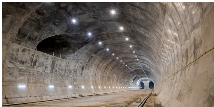
A single span cavern at Victoria Cross Station on the Sydney Metro City & Southwest project
