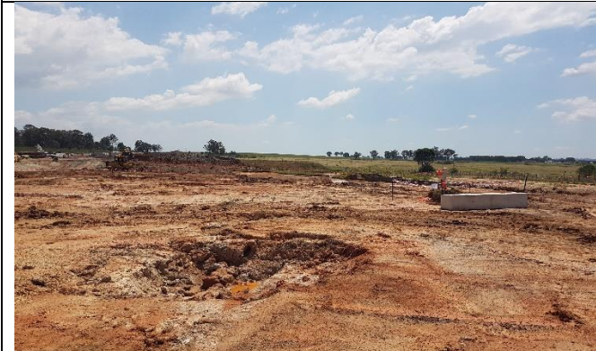
Aerotropolis : View southwest of surface soil stripping and asbestos removal in DSI moderate risk areas.
