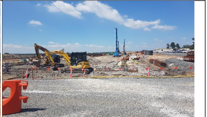
Aerotropolis : View north from entrance of DSI low risk area pile break back, blinding and capping beam FRP.
