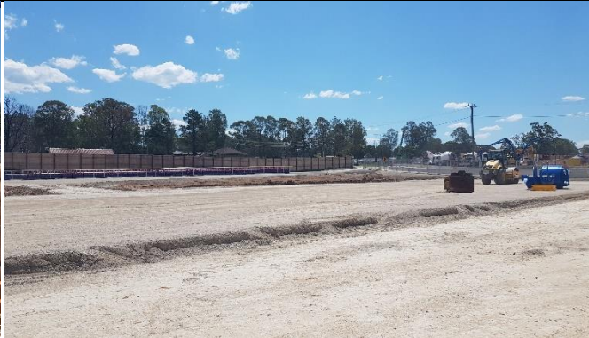
Orchard hills- view south at pilling pad preparation South of Lansdowne Rd .
