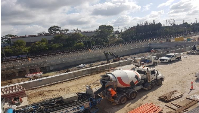
St Marys: View of works to the north showing eastern capping beam and station box excavation
