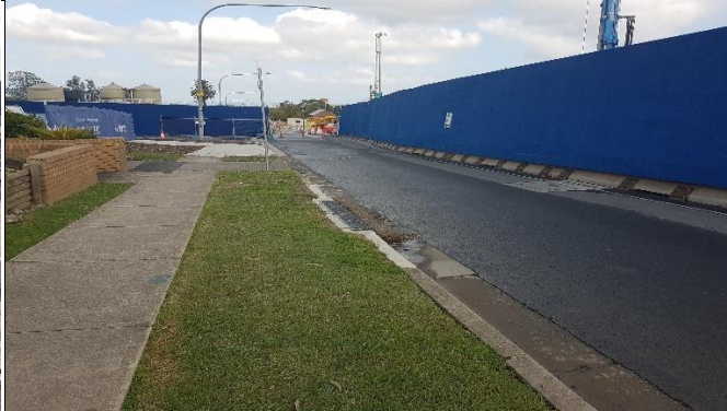
St Marys – Looking west along Station St.
