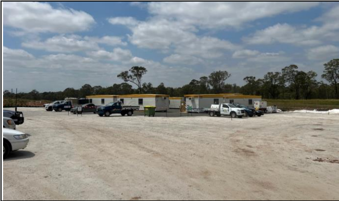
Patons Lane – The site compound is complete
