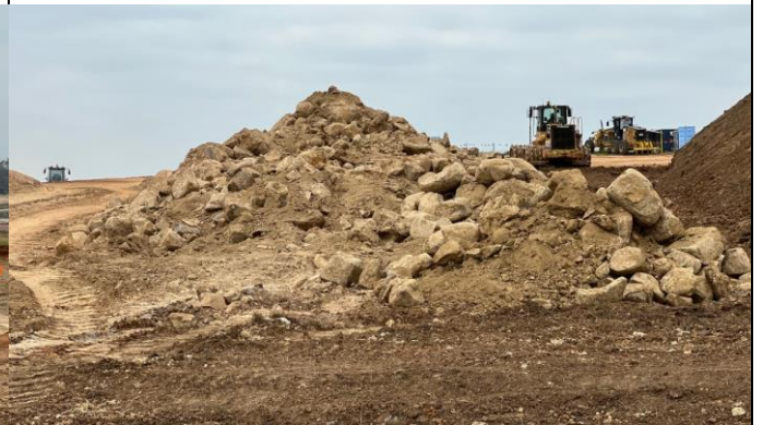
Elizabeth Drive – Rocks and boulders have been stockpiled for use in future ERSED controls
