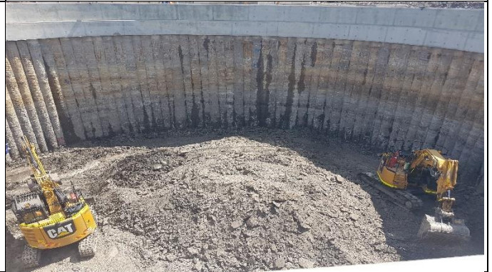
Claremont Meadows view west – Shaft bulk excavation
