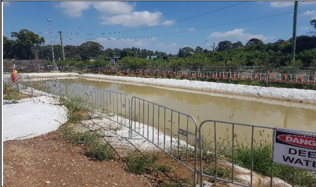
Claremont Meadows – View southwest along Great Western Highway of basin in operation
