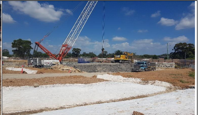
Claremont Meadows view northwest – Shaft excavation spoil.
