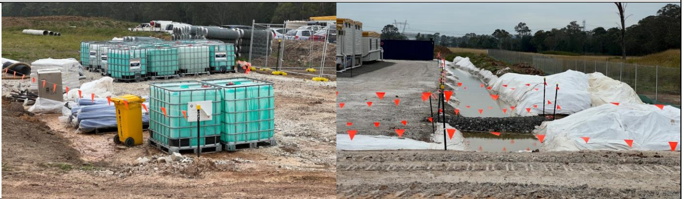
Patons Lane – Polymer compound has been ordered and used on site as an ERSED control
