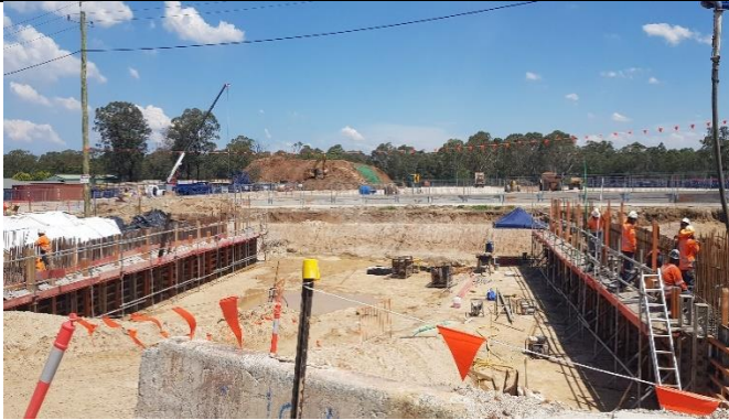
Orchard Hills view south – Capping beam FRP at Lansdowne Rd for bridge over station box.
