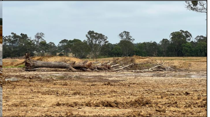
SMF - Trees have been cleared in the SMF with the remained needing ecologist supervision
