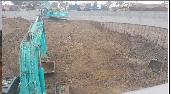
Bringelly Services Facility – Services shaft bulk excavation. Note completed capping beam and upstand
